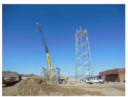
Figure 6. Steel erection of the telecomm tower at Red Bluff Substation.
