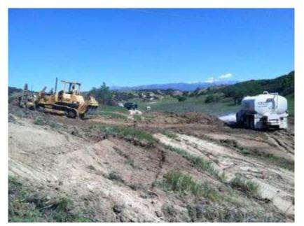
Figure 2. Site clearing at Wire Site 36 near Tower 1101.
