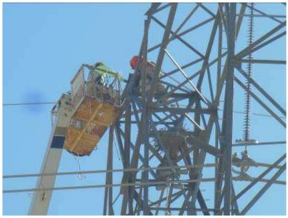
Figure 6. OPGW repair crew working inside 12-ft buffer around active raven nest (note nest in center of photo).
