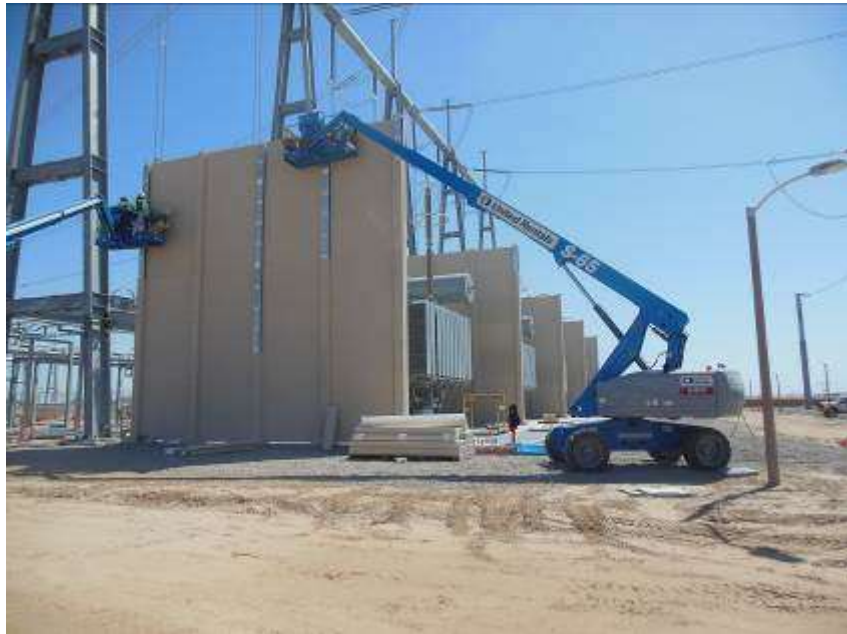
Figure 6. Installing wall panels around the transformers at CRS.
