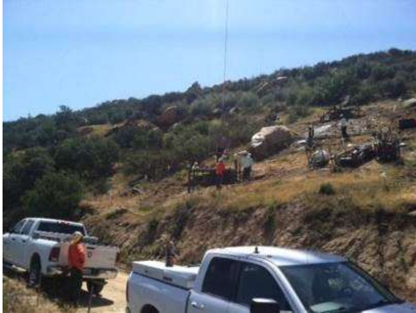
Figure 1. Concrete pouring by helicopter for micropile foundations at Tower 1092.
