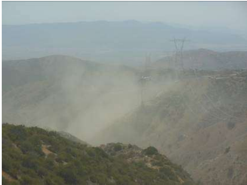
Figure 5. Excessive dust during sky crane operations at Tower 1107.
