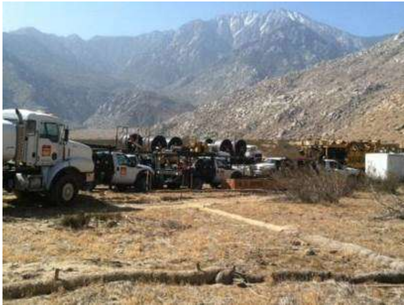
Figure 3. Wire crew set up at the pull site adjacent to Tower1031.
