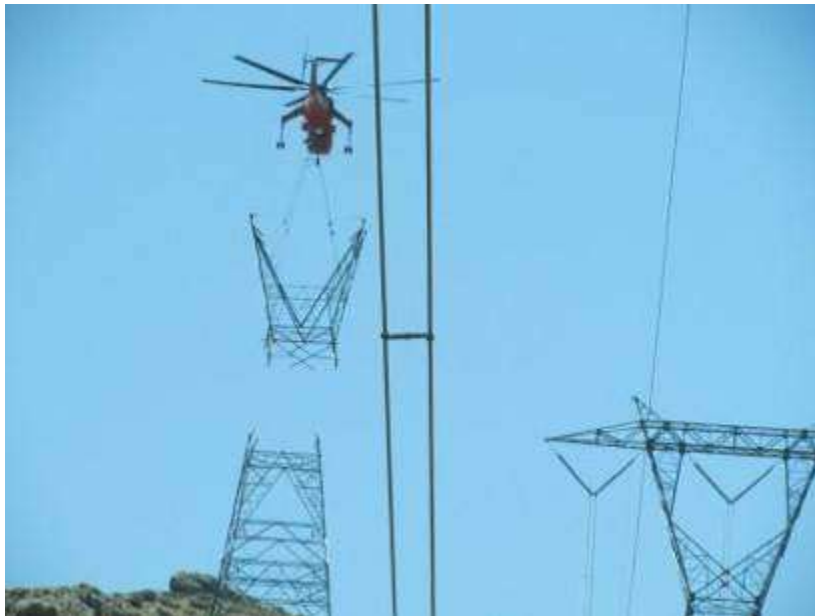
Figure 2. Tower assembly via Skycrane at Tower 1067.
