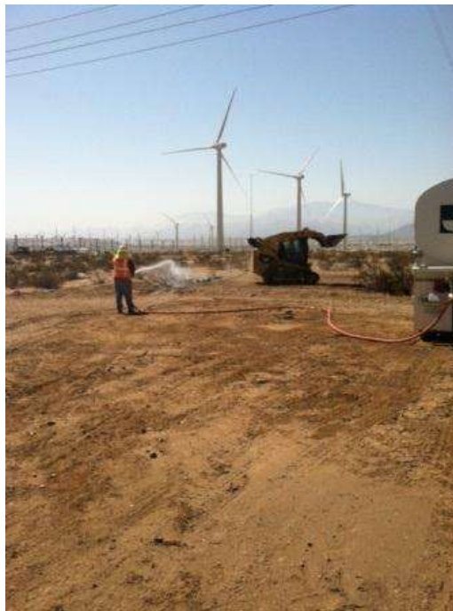
Figure 4. Site stabilization at Tower 1002.
