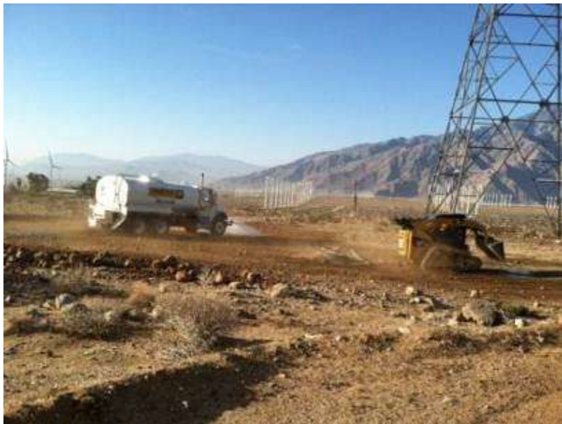
Figure 4. Site stabilization activities at Tower 1005.
