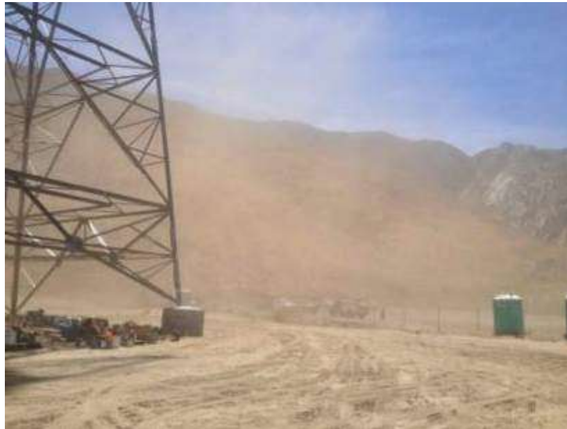
Figure 5. Fugitive dust emissions generated from helicopter activities at HLZ H2A. Photo courtesy of FRED
