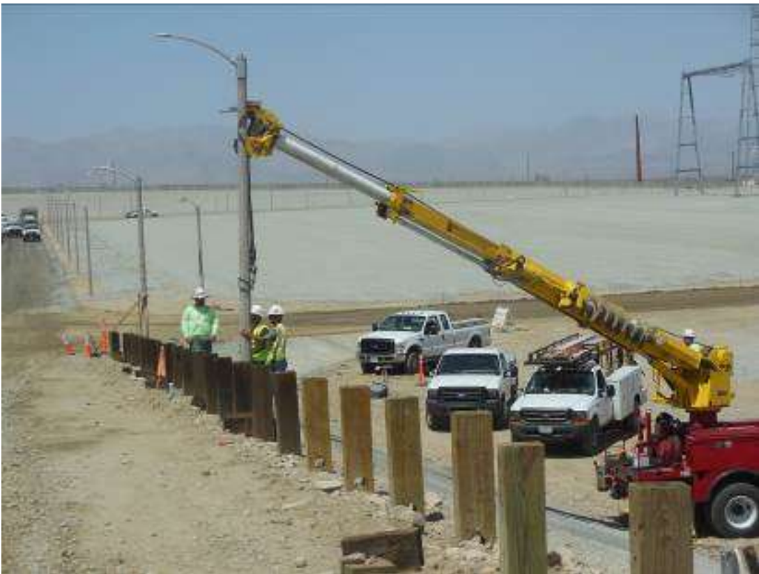
Figure 8. Installing lights at Red Bluff.
