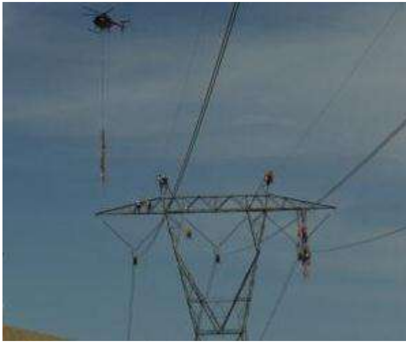
Figure 3. Helicopter related wire stringing activities at Tower 1029. (Photo courtesy of FRED)
