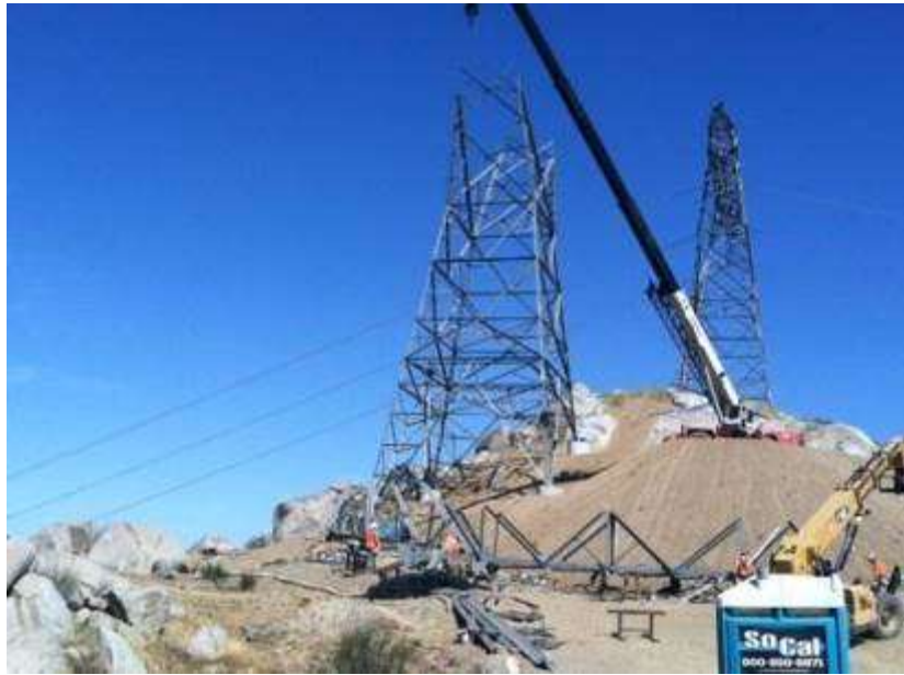
Figure 3. Tower assembly at Tower 1127.
