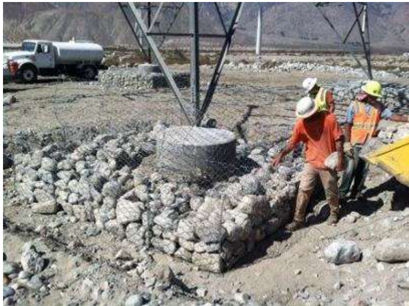
Figure 2. Gabbion basket installation at Tower 1018
