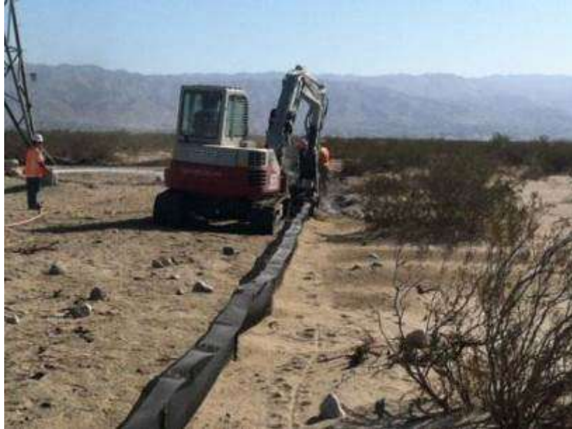
Figure 1. CVFTL fencing removal at Tower 2012.
