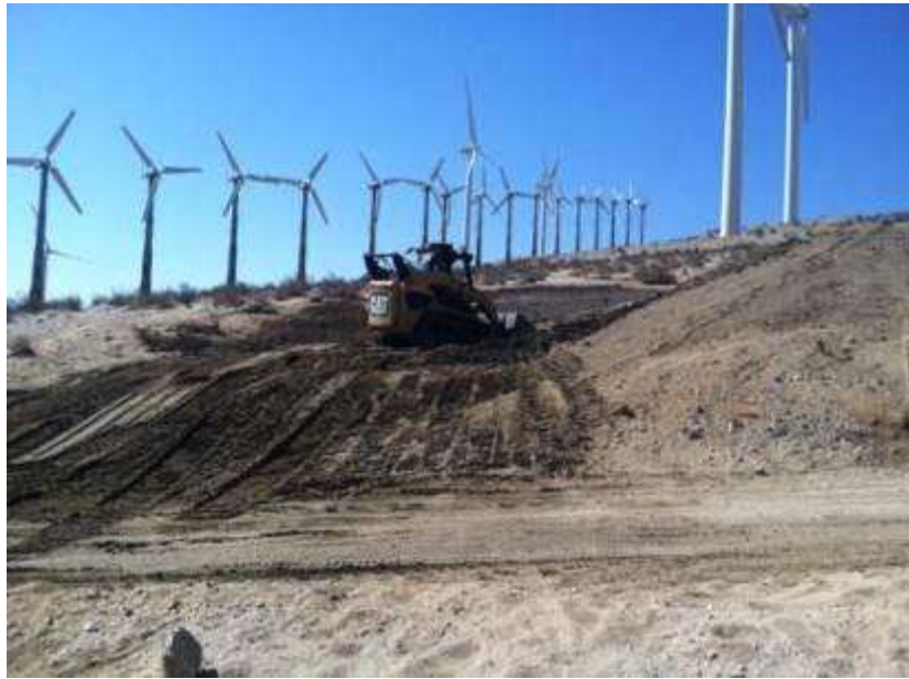
Figure 5. Site stabilization at Tower 1011.
