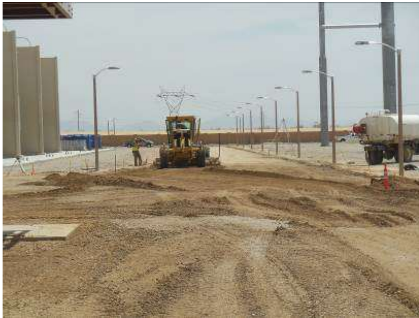
Figure 7. Installation of interior road base at CRS.
