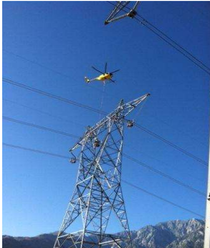
Figure 4. Installation of wire spacers at Tower 1030.
