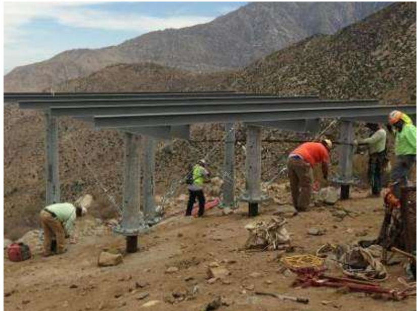
Figure 6. Permanent platform installation at Tower 1040.
