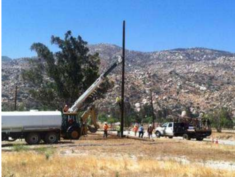
Figure 1. Guard pole installation near Tower 1078.
