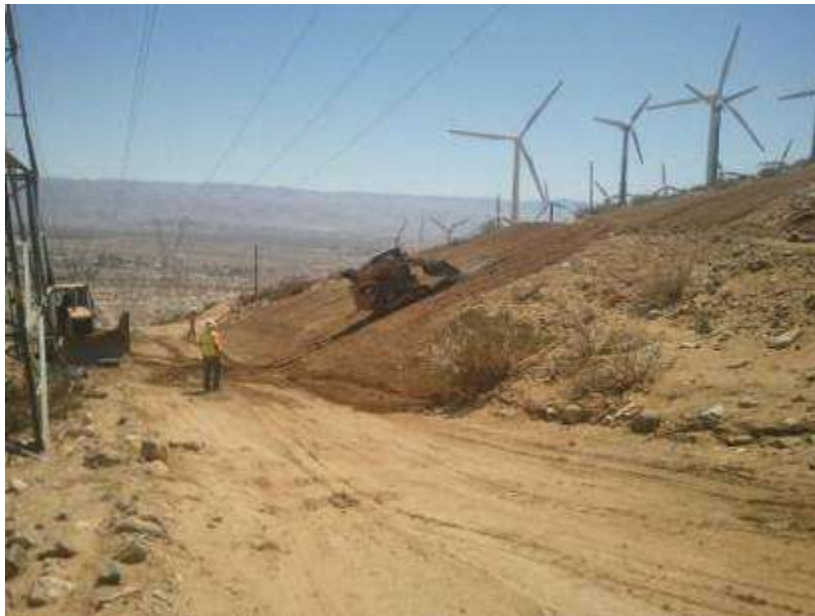
Figure 2. Site stabilization at Tower 1012 (Photo courtesy of FRED).
