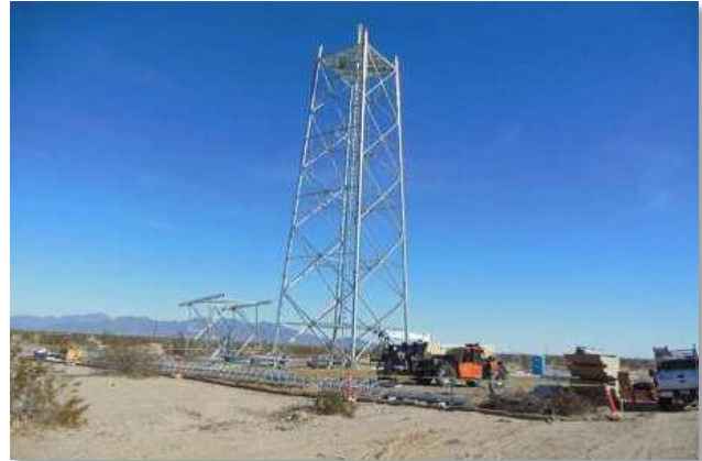
Figure 20. Erection of the telecom tower at the Desert Center site.
