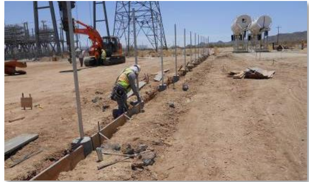
Figure 18. Fencing installation at Series Capacitor site.
