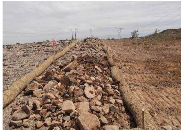
Figure 3. Stockpiled Desert Pavement clearly defined at Tower 2529.
