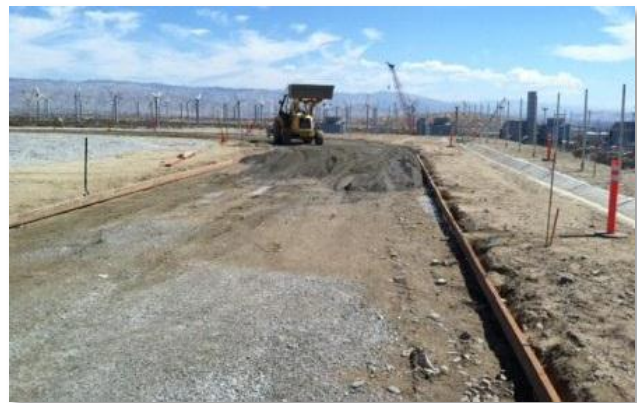
Figure 16. Paving activities within the expansion area at the Devers Substation.
