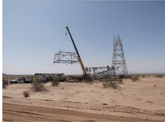
Figure 2. Assembly of Tower 2649 and CR1-2W.
