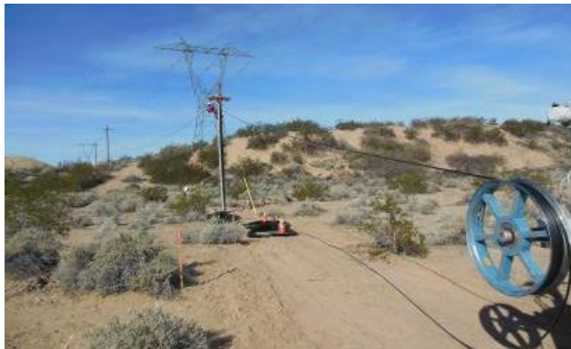
Figure 19. Overhead ground wire pulling operations along the Southeast Telecomm Line.
