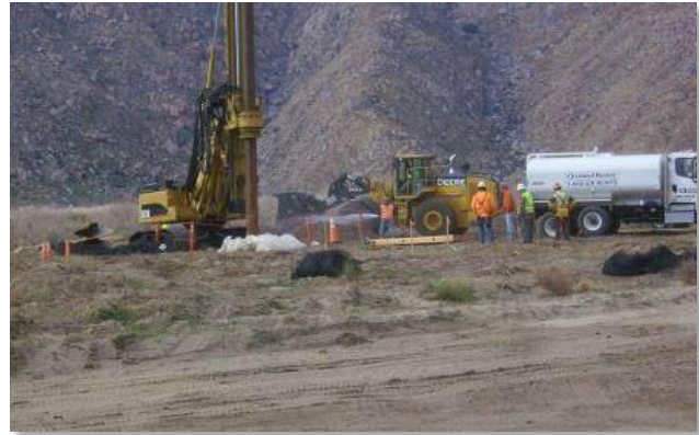
Figure 5. Conventional foundation drilling at Tower 1061.
