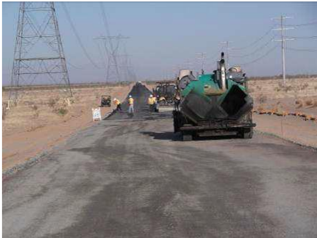
Figure 12. Road paving activities along the primary CRS access road.
