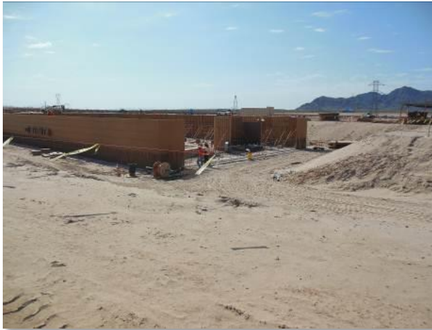
Figure 11. Construction of the MEER building at CRS.
