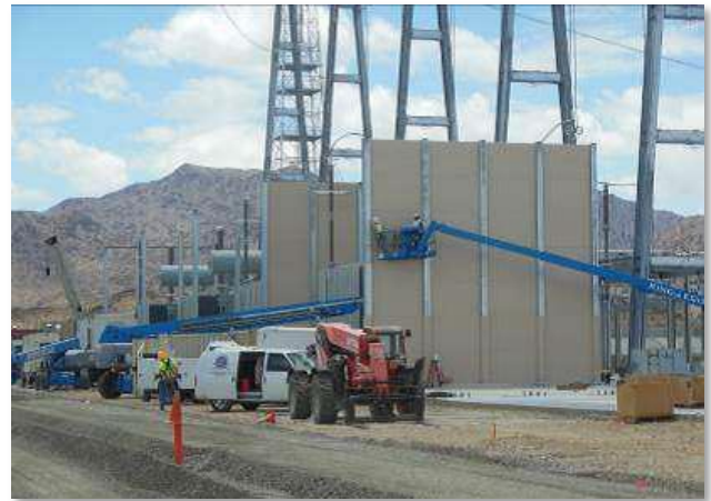
Figure 14. Installation of transformer panels within the Red Bluff Substation
