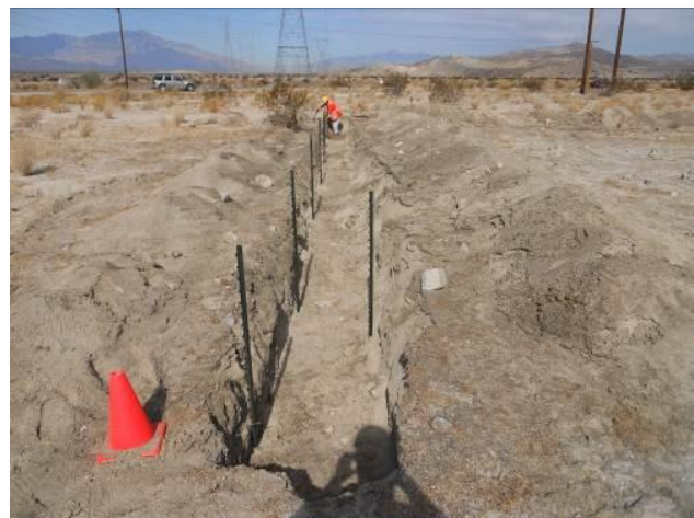
Figure 4. Installation of CVFTL/FTHL exclusionary fencing at Tower 2211.
