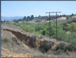
Maraschino Loop West. Replace single-circuit wood poles with new single-circuit steel poles.
