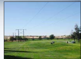
Existing 115 kV subtransmission line through the Sun Lakes Community.
