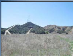
Looking south toward the proposed site for the El Casco Substation on the Norton Younglove Reserve. (Existing SCE towers are shown in the background.)
