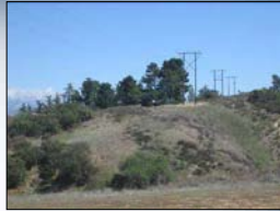
Existing single-circuit wood poles going into Maraschino Substation. These will be replaced with new single-circuit steel poles.
