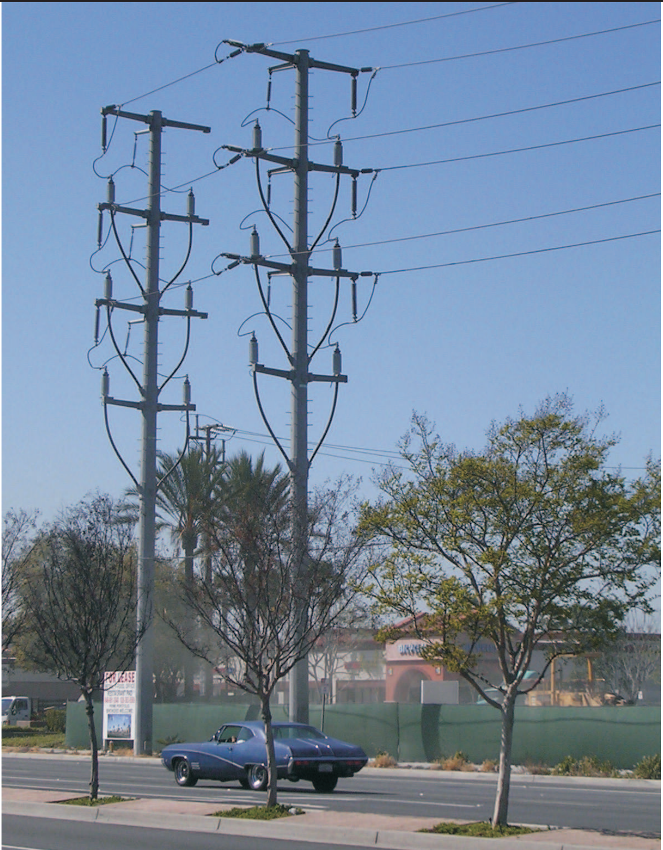
Figure C-5 Example of Double-Circuit 66 kV Riser Poles
