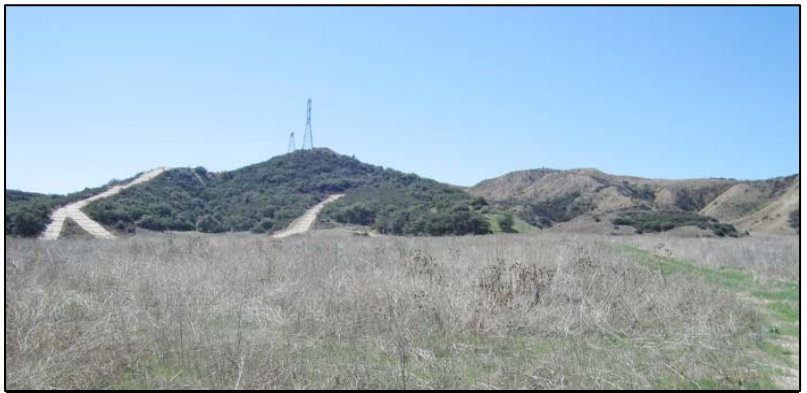
Looking south towards the proposed site for the El Casco Substation on the Norton Younglove Reserve (existing SCE towers are shown in the background)
