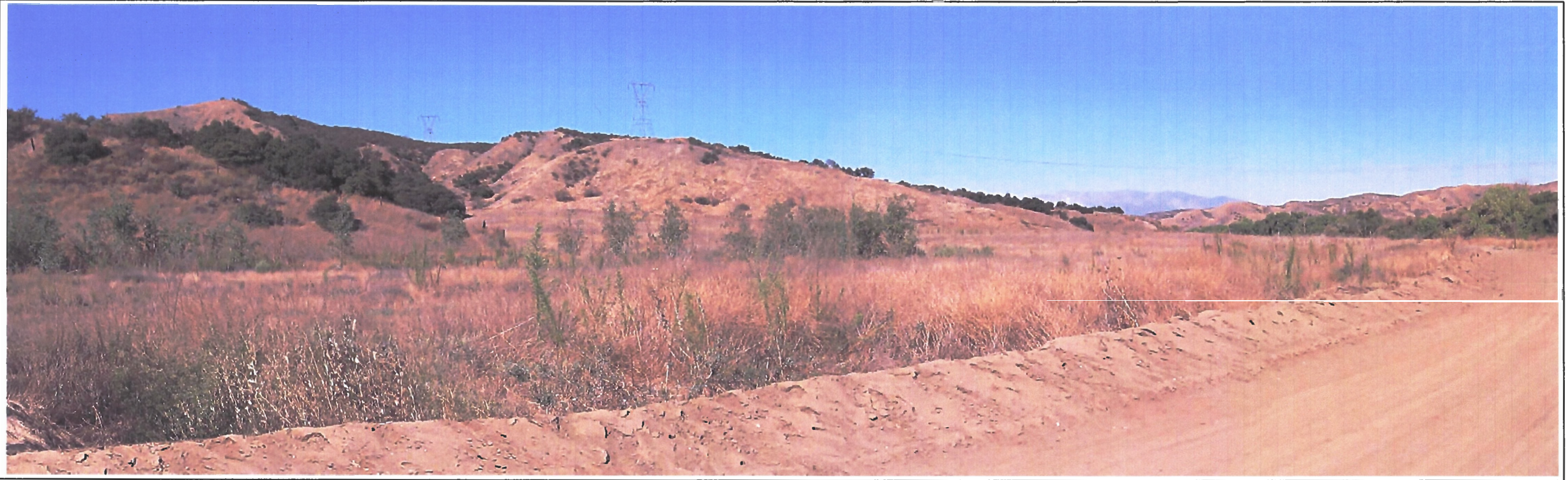
Existing view of El Casco Substation Site from Key Viewpoint #1.
