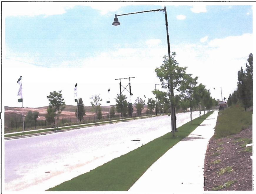
Existing view of 115 kV subtransmission line from Key Viewpoint #6.
