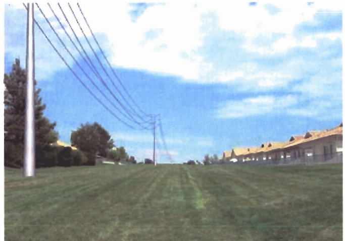
Figure 3B. Looking East from Highland Springs Road Proposed 115 kV Subtransmission Line
