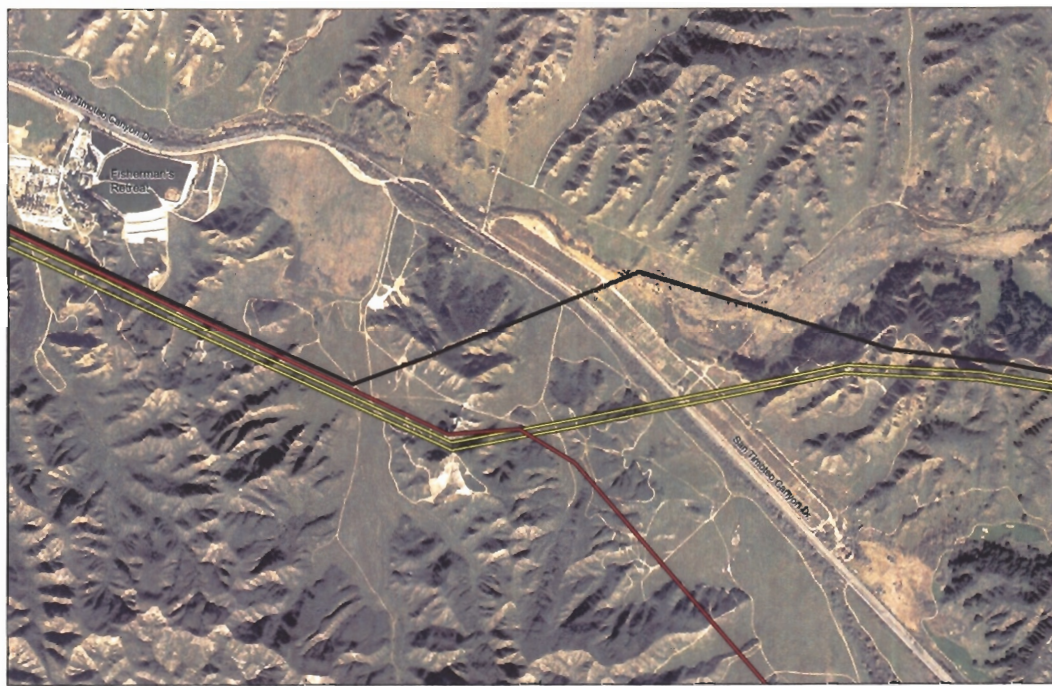
Existing Site for Proposed El Casco Substation
