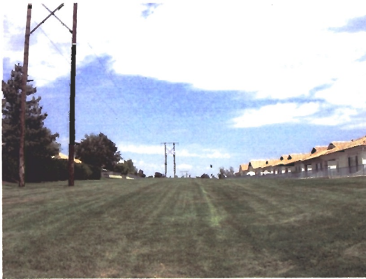
Existing view of 115 kV subtransmission line looking east from Highland Springs Road (Key View 5)
