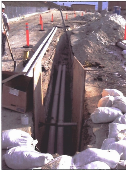
1. Grade the site and install underground conduits
