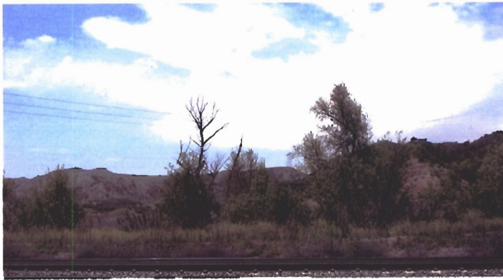
Existing view of El Casco Substation Site from San Timoteo Canyon Road (Key View 3)
