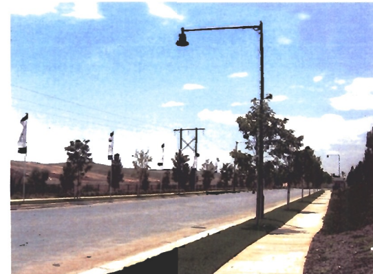
Existing view of 115 kV subtransmission line looking west from Highland Springs Road (Key View 6)
