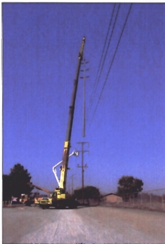
3. Set new pole in place
