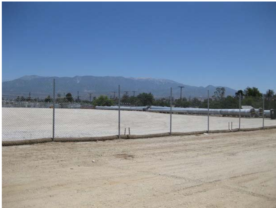
Figure 5: Transmission towers are being stored at the Maraschino Substation Laydown Yard. The east border fence which separates the yard from the vegetated portion of the property is beyond the stacked towers. The photograph faces northeastward.
