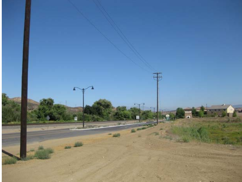
Figure 3: On San Timoteo Road, the existing utility line was placed underground (past the second pole visible) as part of road improvement connected with the new development on the right. The fiber optic cable will be placed within conduit in place. The photograph faces westward.
