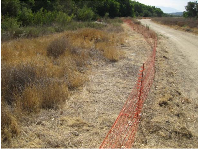
Figure 1: Exclusion fencing was placed around smooth tarplant populations adjacent to planned culvert installation at one location on the El Casco Substation access Route. The culvert installation will be the next construction activity at the substation. It will begin after September 1, 2009. The photograph faces eastward towards the substation site. San Timoteo Creek is to the left. The realigned access route will be immediately to the right of the existing road.
