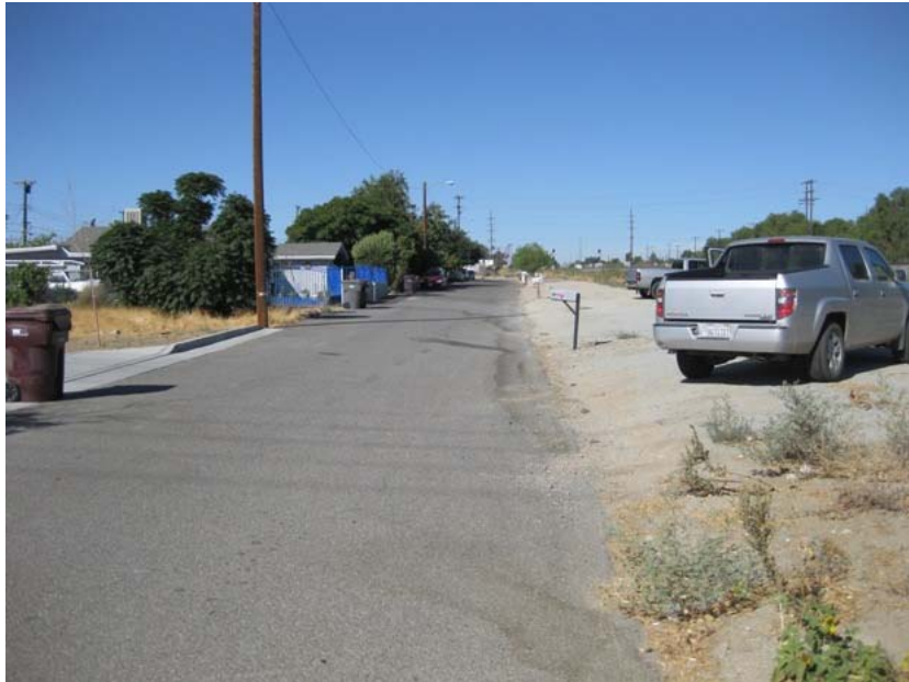
Figure 1: SCE will be submitting a request to enter the Banning Substation during substation construction work via the alleyway on the north side of the substation called John Street. The eastern access to John Street involves a paved section with approximately six occupied homes along a street approximately 20 to 24 feet wide. Vehicles often park on the curb side of the street on the left. The photograph faces westward.
