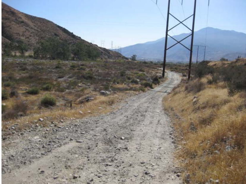
Figure 2: The Banning Shoo-fly FOC route is entirely within natural and rangeland habitat. It stretches from the San Gorgonio Creek (in the distance) west for two and one-half miles to Sunset Road. It crosses grasslands and brush-covered hillsides and ravines. Most of the route is accessible by existing SCE dirt roads. In areas not accessible by roads, crews will hand carry materials to the poles, using pile-climbing for installation. The photograph faces southeastward.
