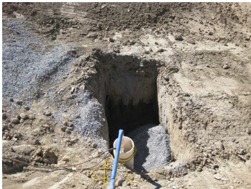
Figure 6: Water is currently being continually pumped out of the excavated pit.
