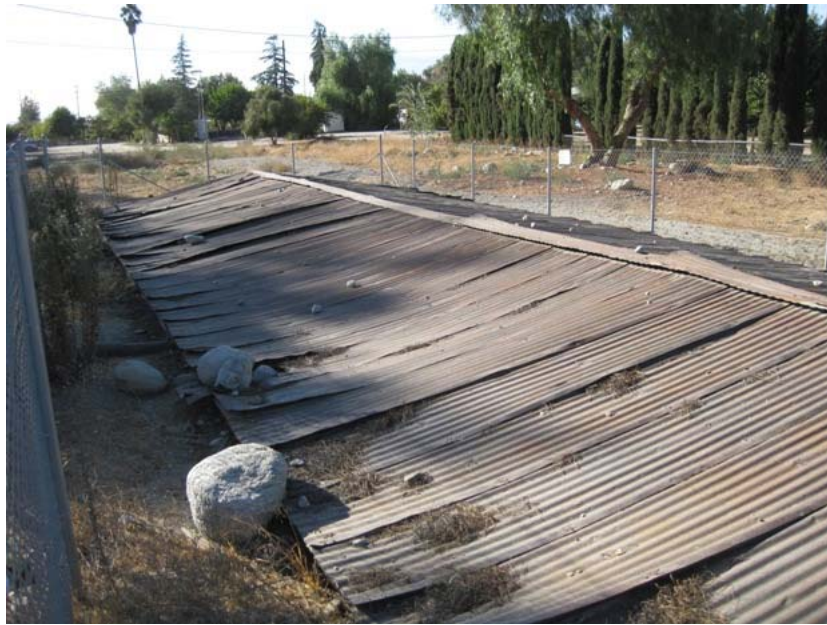
Figure 5: The source of the contaminated water in the ruptured pipeline is this abandoned underground storage tank. It is in a field on the north side of Colton Street. The photograph faces westward. The Mentone Substation is located a few hundred feet in the distance.
