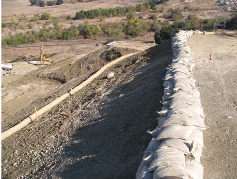
Figure 2: Straw wattling was placed on the cleared hillsides to prevent erosion, and sand bags were placed near the top of the terraced area to direct runoff water away from the cleared hillsides. No significant erosion occurred on these terraced slopes during the subject week. The photograph faces northward.
