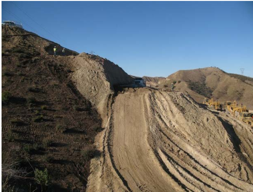
Figure 3: Excavation of the lower terraces at the El Casco Substation site is now being accomplished with scrapers. The photograph is shows the lower portion of the western ridge, and faces southward.
