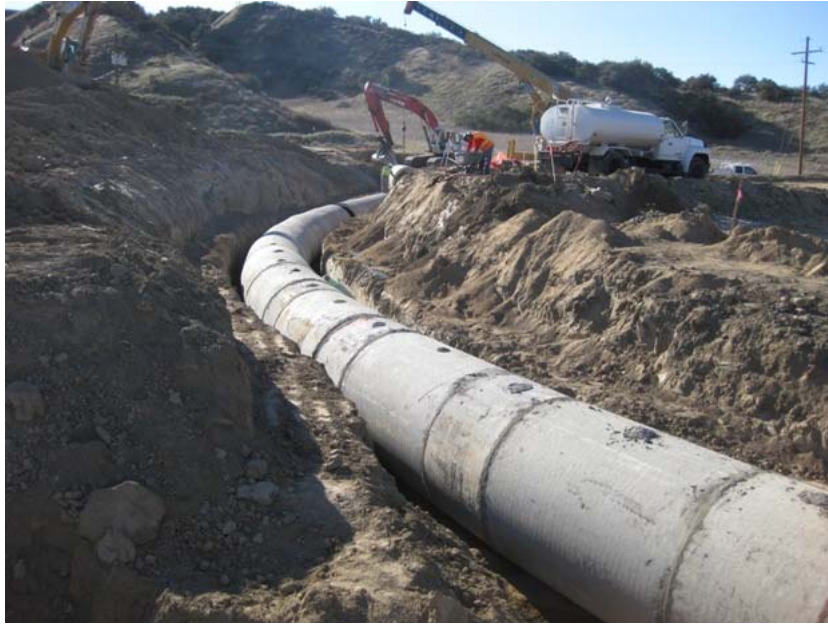
Figure 1: At El Casco Substation, a system consisting of V-ditches and concrete conduit (in photo) is being built to shunt run-off water from higher ground to the south and southwest of the station site around the western side of the station pad to San Timoteo Creek. The photograph faces southwestward.
