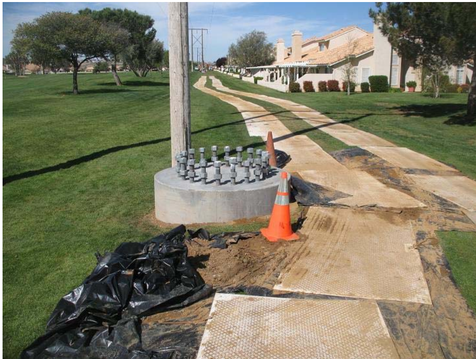
Figure 4: View of completed pole foundation. The photograph faces westward.
