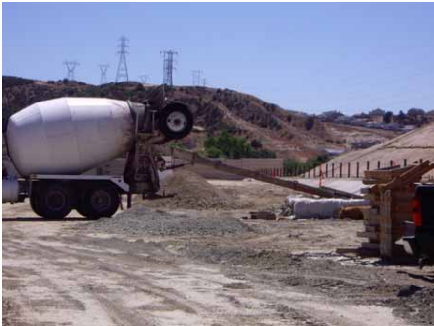
Figure 4: Cement truck using wash-out basin. This photograph is taken facing east.
