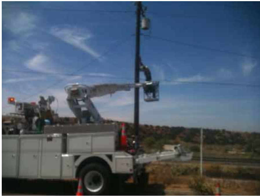
Figure 5: SCE fiber optic crew installing cable.
