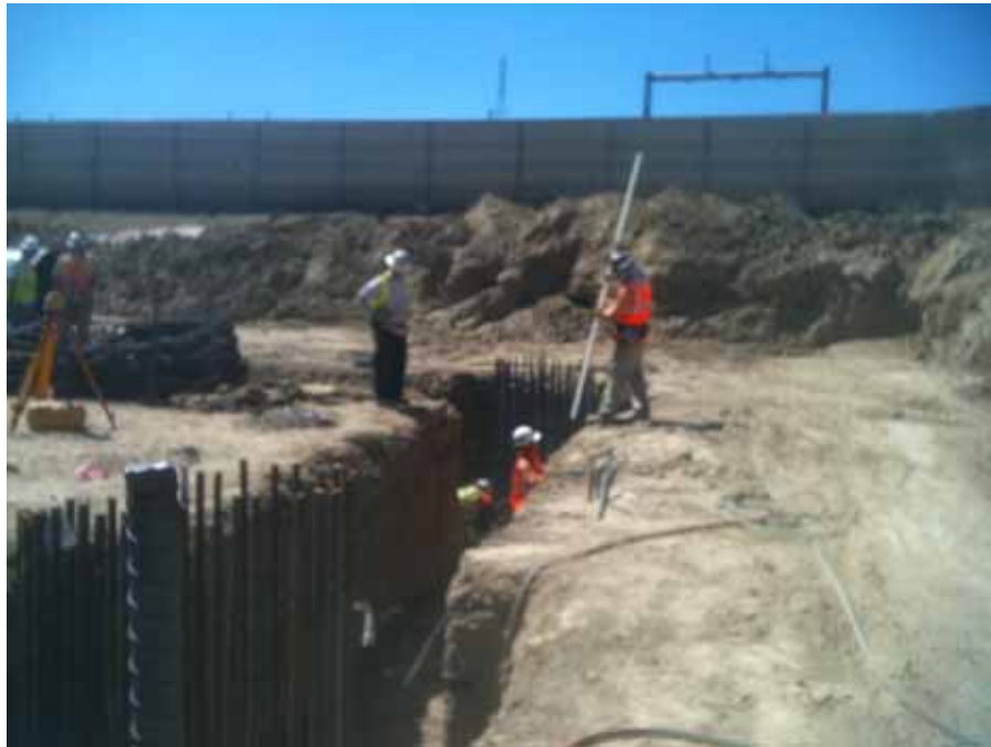
Figure 4: At the El Casco Substation site, work advanced on tower pads.
