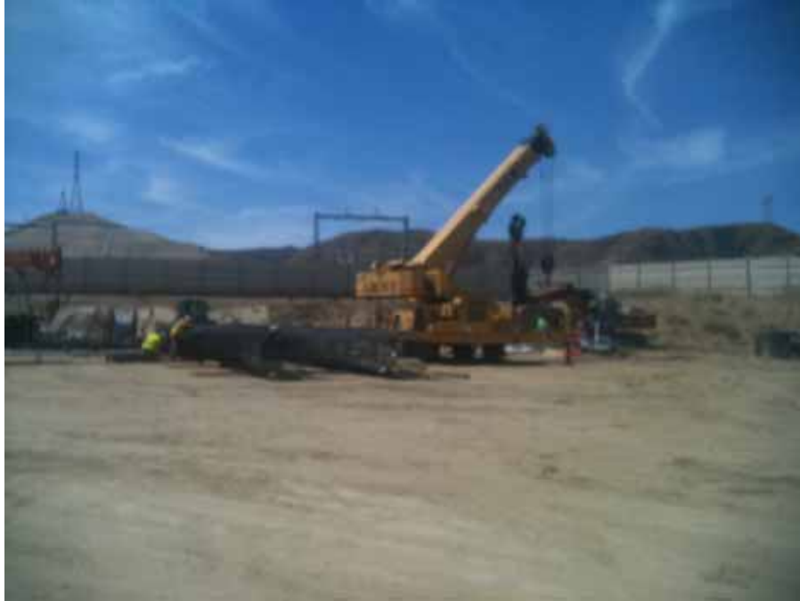
Figure 3: At the El Casco Substation site, work advanced on tower pads.
