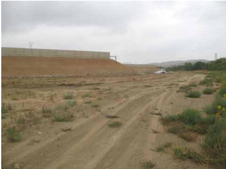
Figure 2: At the El Casco Substation site, a water truck sprays water on the spoil spreading area.
