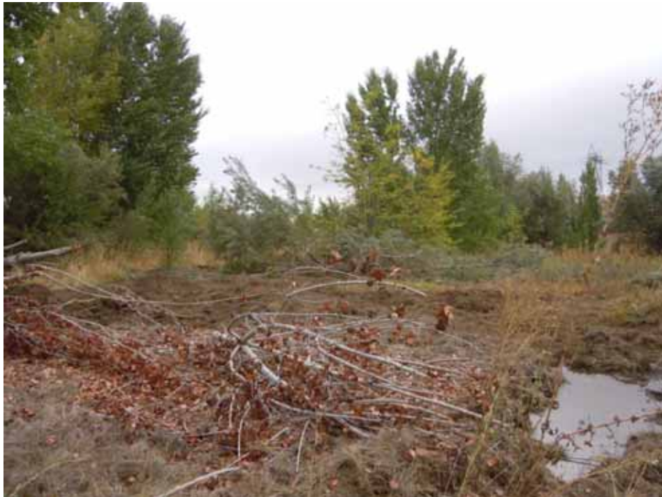
Figure 4: Outside the El Casco Substation site along San Timoteo Canyon Road, vegetation removed with the stolen excavator.
