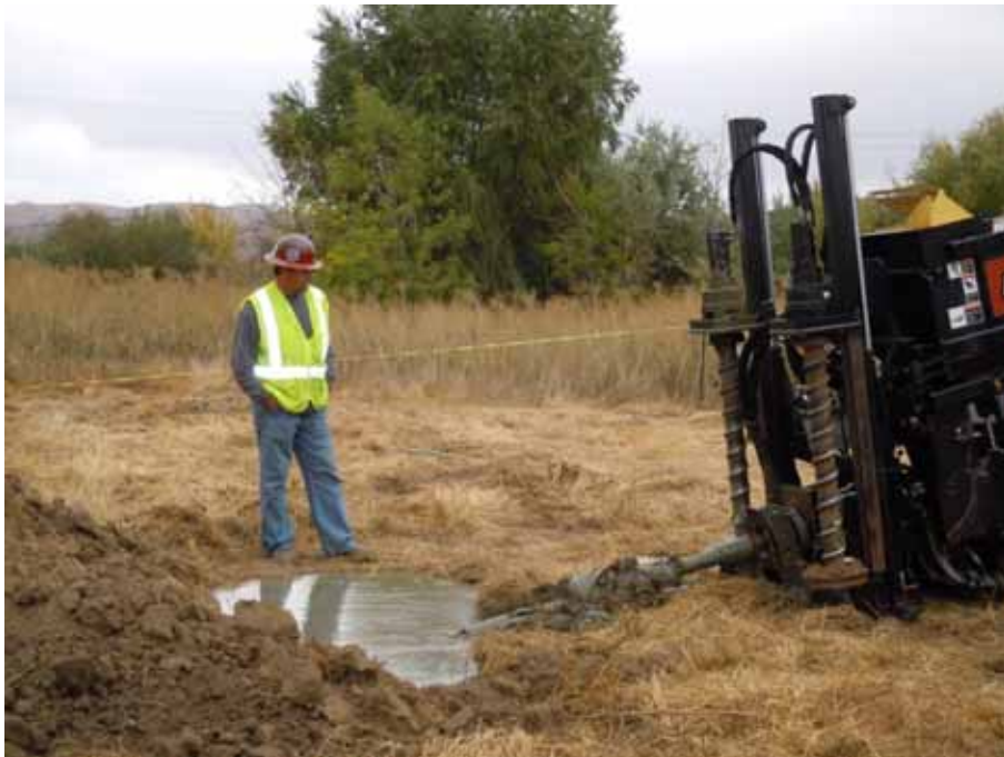
Figure 2: Outside the El Casco Substation site, HDD work began.
