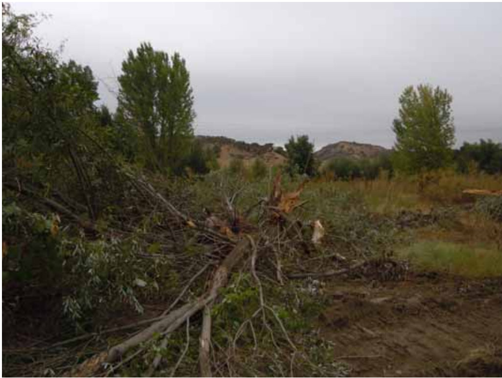
Figure 5: Outside the El Casco Substation site along San Timoteo Canyon Road, a tree broken with the stolen excavator.
