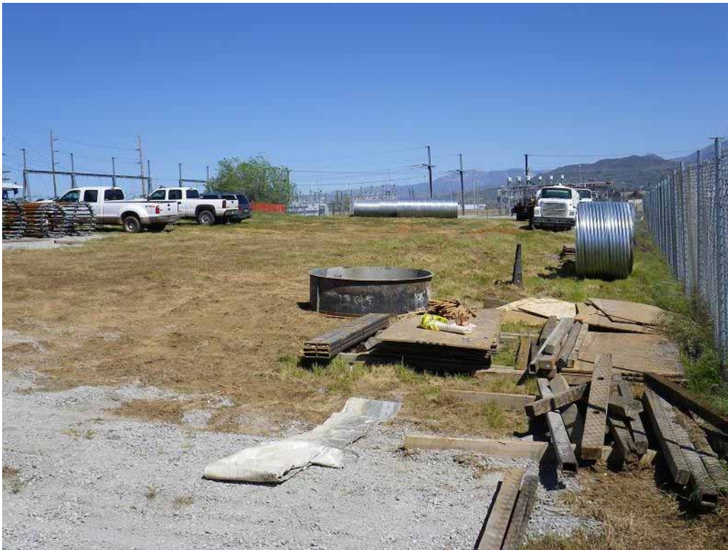
Figure 4: Recently expanded storage yard at the Maraschino Substation.
