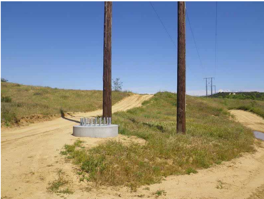
Figure 2: View of completed pole foundation on Segment 7. The photograph faces east.
