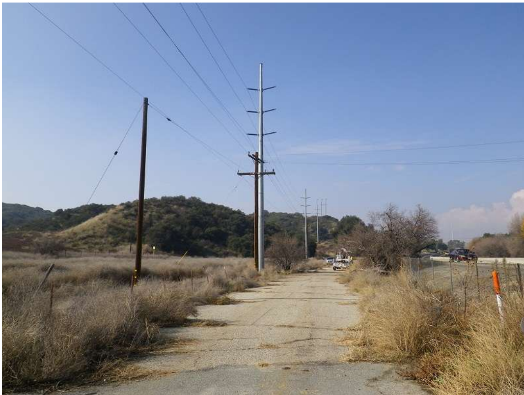
Figure 4: View of recently installed poles along Segment 7. The photograph faces west.
