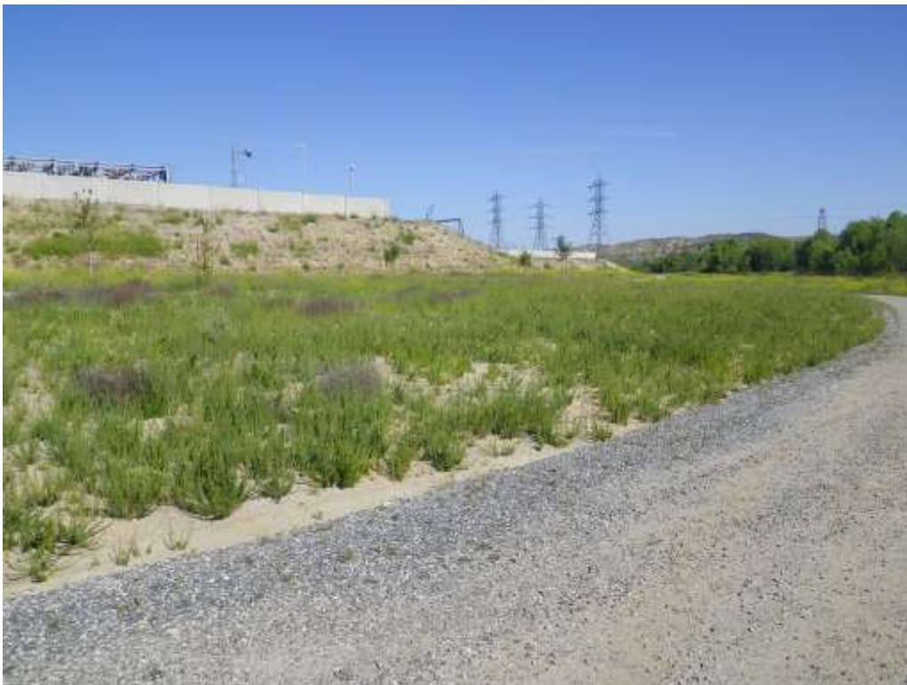
Figure 2: View of restoration area just north of the El Casco Substation. The photograph faces northwest.
