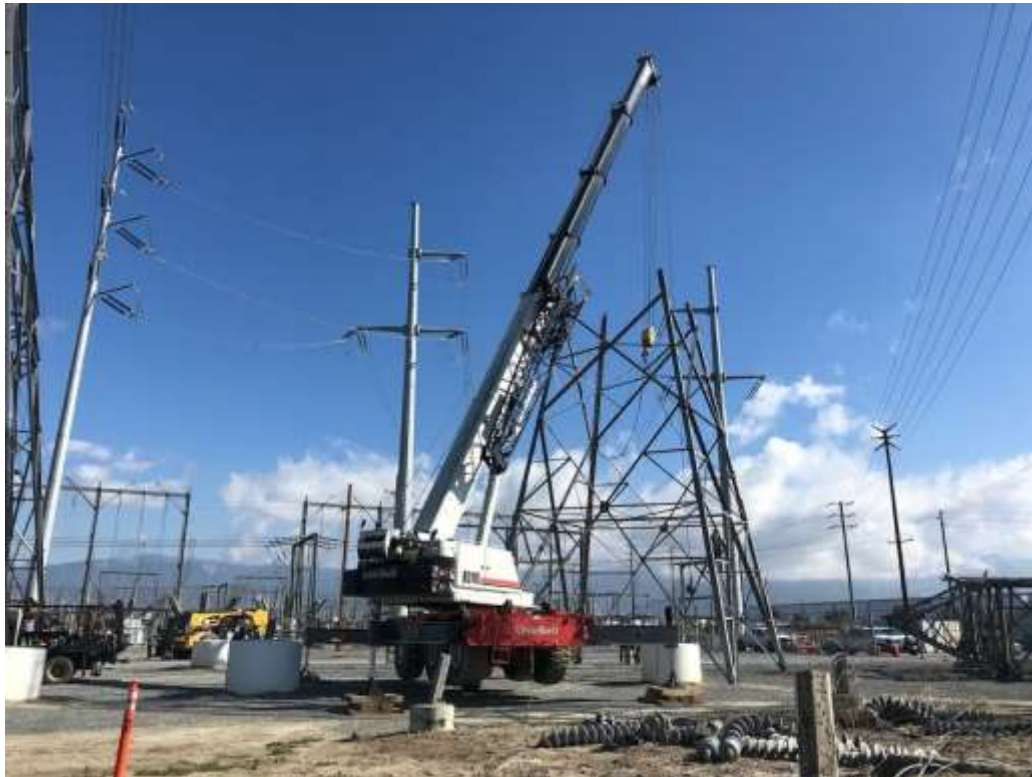
Photo 2 – Tower wreck-out at Construction Area 1X26, Segment 1 (March 26, 2020).
