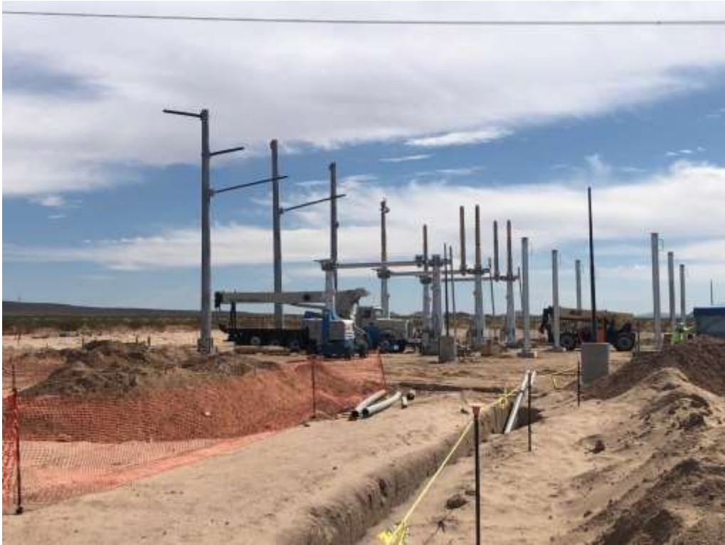
Photo 1: Progress at Ludlow Midline (October 6, 2021).
