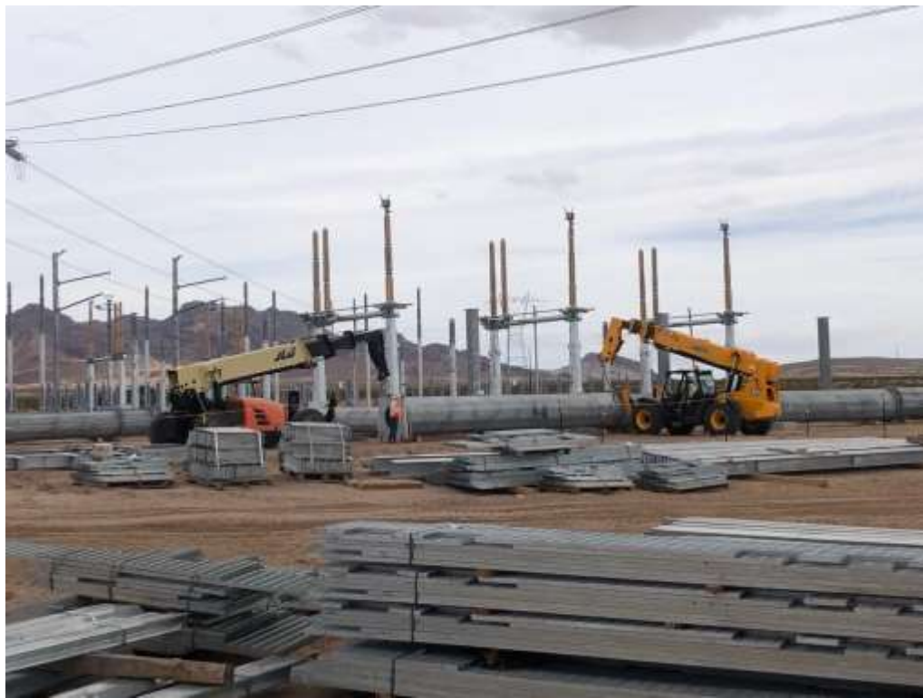
Photo 2: Progress at Ludlow Midline (October 25, 2021).
