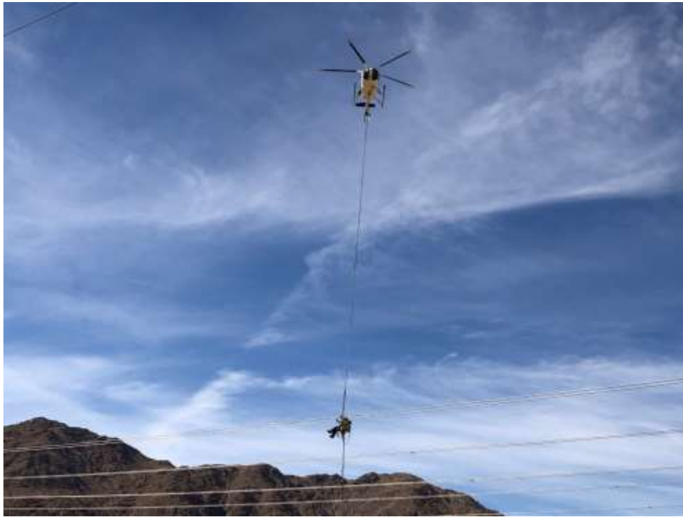
Photo 3: Pulling wires near Barstow Repeater (October 20, 2021).
