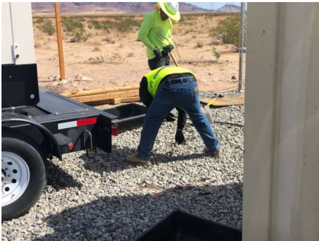
Photo 6: Analysis of generator spill from October 4 (October 6, 2021).
