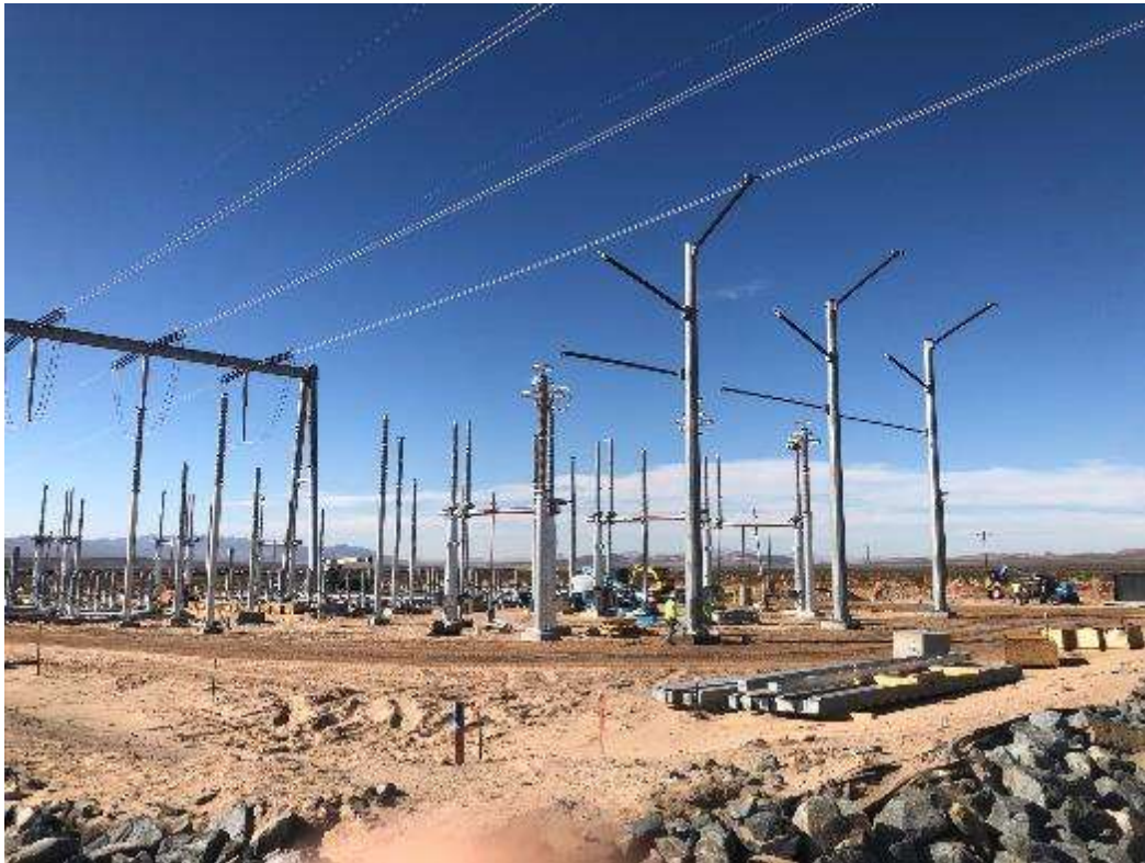
Photo 3: Assembly of platform base and pedestals at Ludlow Series Capacitor (November 23, 2021).
