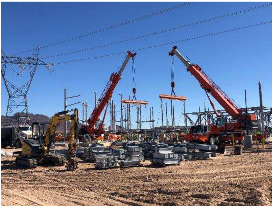
Photo 4: Assembly of platform base and pedestals at Ludlow Series Capacitor (November 30, 2021).
