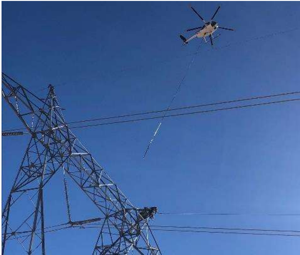
Photo 5: Wire pulling and tower modifications (November 3, 2021).
