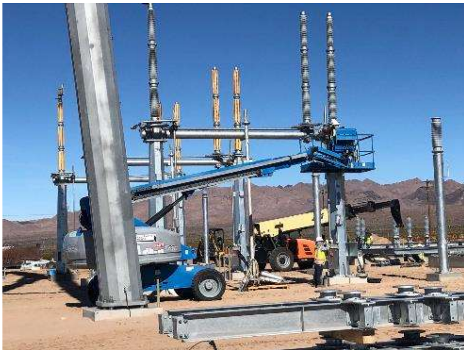
Photo 2: Installing A Frame Interset Structure, Ludlow Midline (November 10, 2021).
