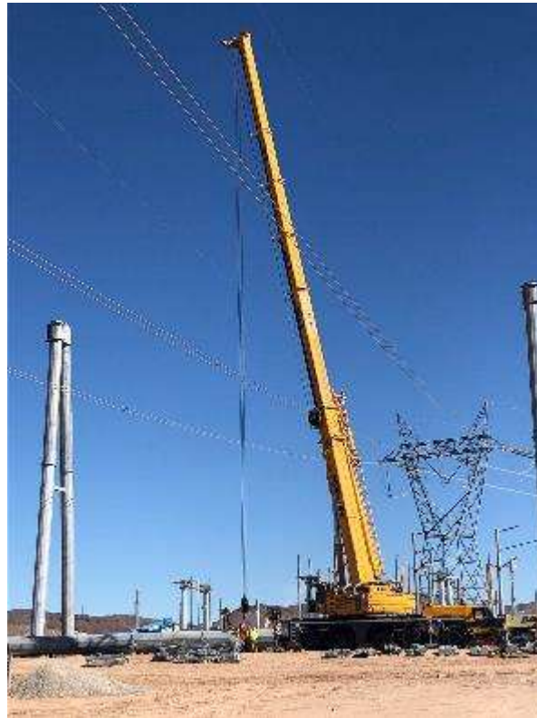
Photo 1: Installing A Frame Interset Structure, Ludlow Series Capacitor (November 3, 2021).
