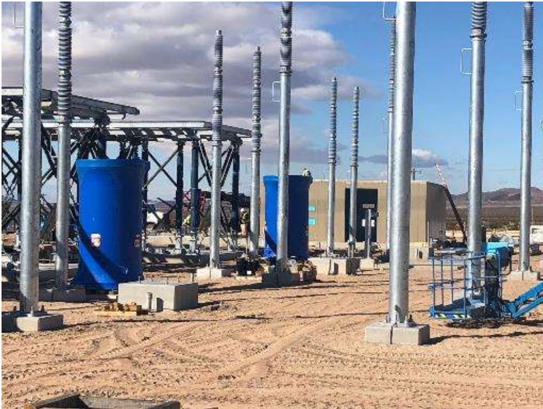
Photo 3: Assembly of MEER building at Ludlow Series Capacitor (December 27, 2021).
