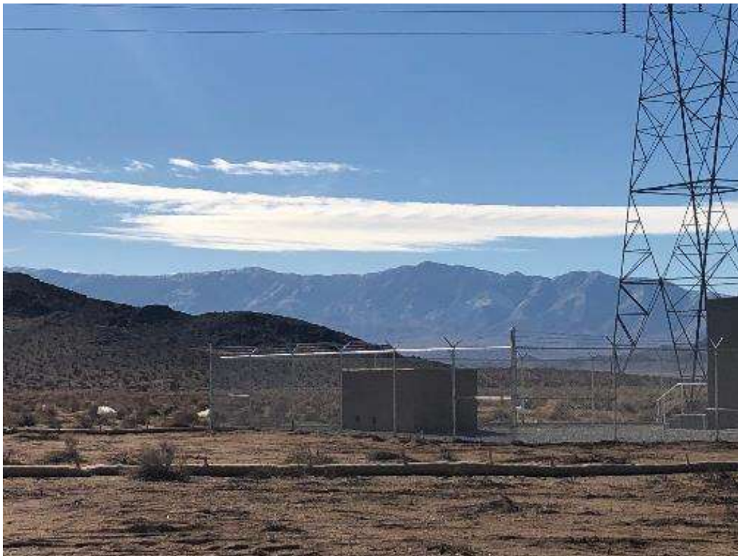
Photo 4: Completed construction along Lugo-Mohave transmission line, Barstow Repeater (December 27, 2021).
