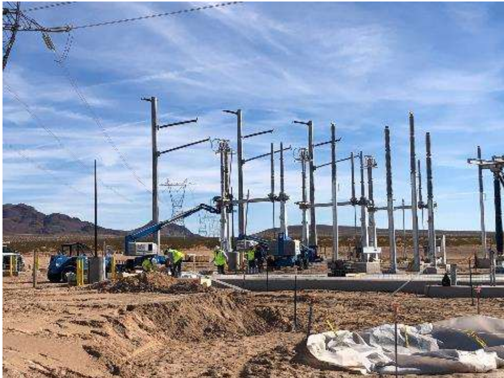
Photo 2: Sack and patch pier foundations, Ludlow Series Capacitor (December 20, 2021).
