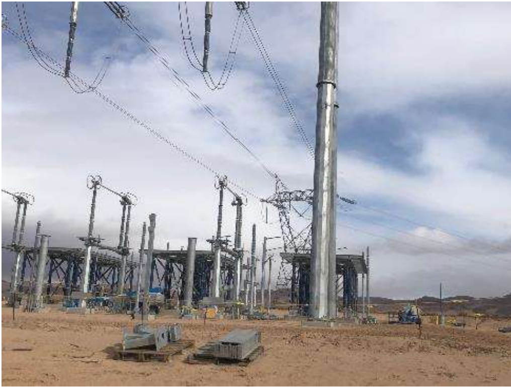
Photo 1: Sack and patch pier foundations, Ludlow Series Capacitor (December 14, 2021).
