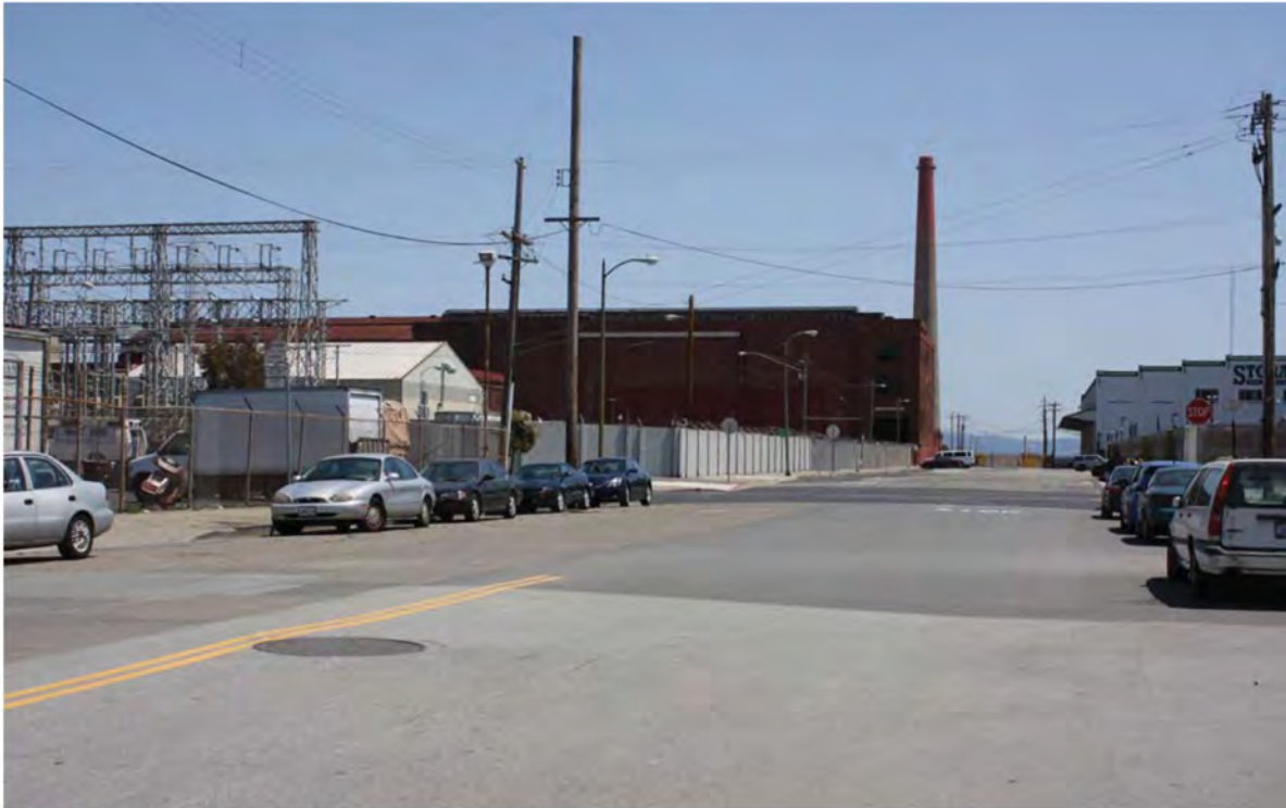
3. 23rd Street at 3rd Street looking northeast
