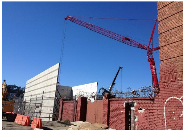
Figure 7. Installing wall panels of GIS building at Potrero Switchyard, October 29, 2015
