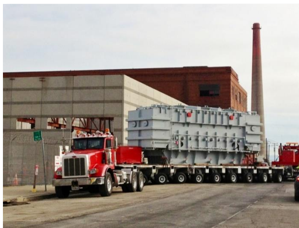
Figure 12. Transformer being delivered to switchyard, December 17, 2015
