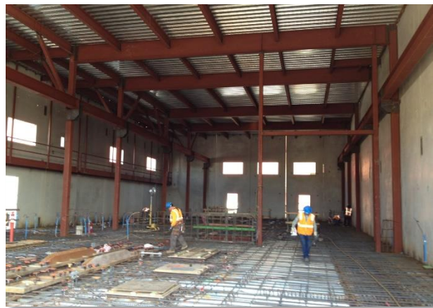
Figure 9. Inside GIS building prepping for concrete floor pour, February 24, 2016
