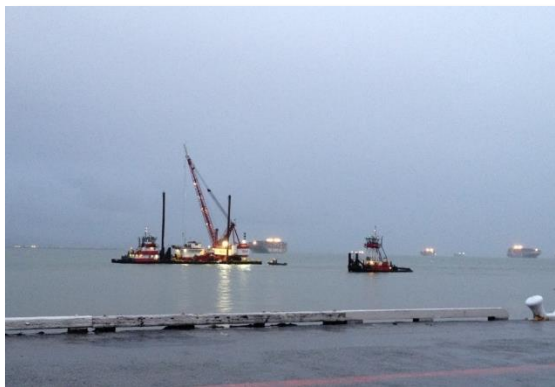
Figure 24. Manson dredging for rock and debris off Pier 30-32, December 17, 2014
