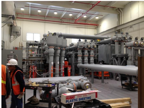
Figure 10. Installation of equipment in GIS building, July 12, 2016
