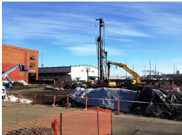
Figure 3. Potrero Switchyard soil displacement work, February 26, 2015
