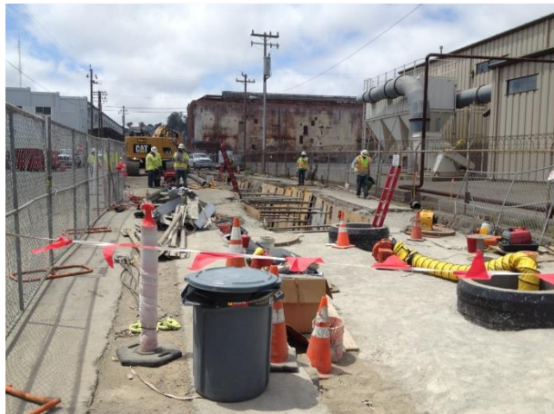
Figure 22. Duct Bank South installation of conduit on 23rd Street, May 15, 2015
