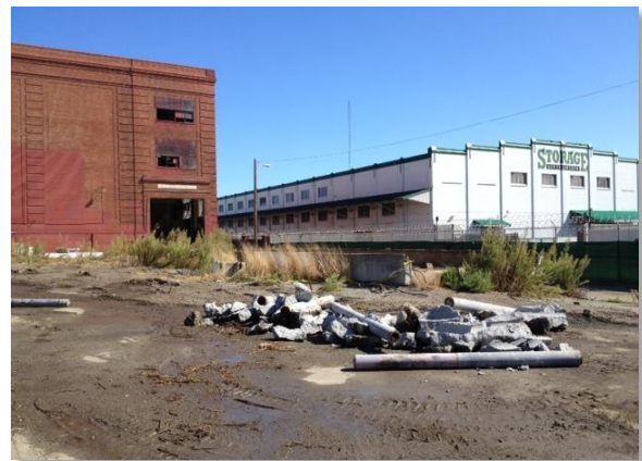
Figure 2. Potrero Switchyard demolition and debris removal, October 9, 2014
