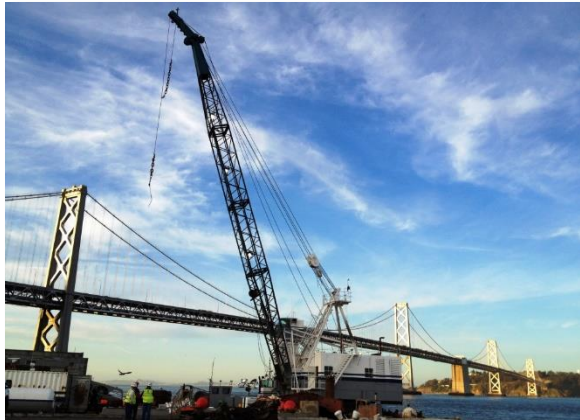
Figure 16. Vortex set up at Pier 30-32 to aid HDD operations, February 26, 2015
