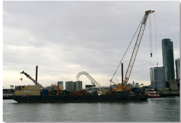
Figure 25. Cable-laying barge, June 10, 2015
