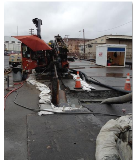
Figure 17. HDD South on 23rd Street, November 20, 2014
