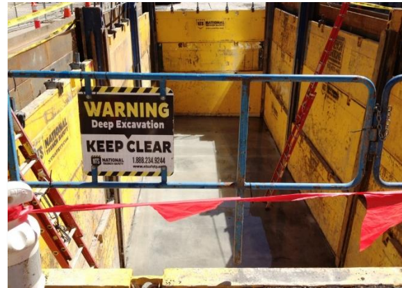
Figure 19. Vault pit shored on Spear Street, March 25, 2015
