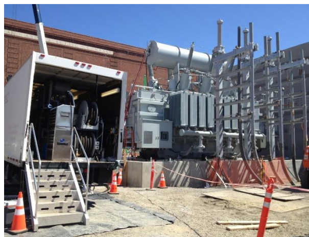
Figure 13. Crews working on assembling the transformer, March 31, 2016
