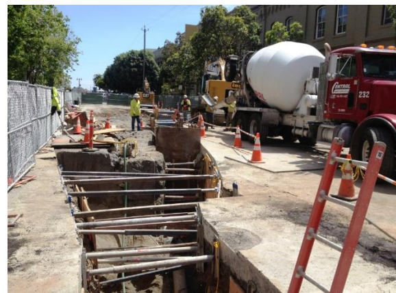
Figure 21. HDD to duct bank transition on Spear Street, April 28, 2015
