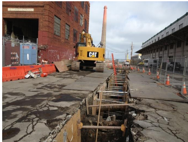
Figure 23. Excavating for Duct Bank South on 23rd Street, September 22, 2015
