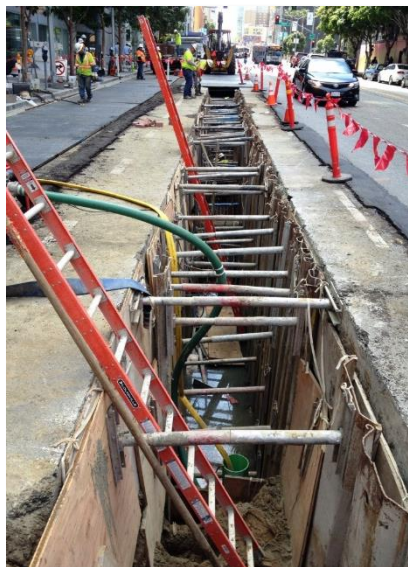
Figure 18. Setting rebar in duct bank on Folsom Street, April 1, 2015
