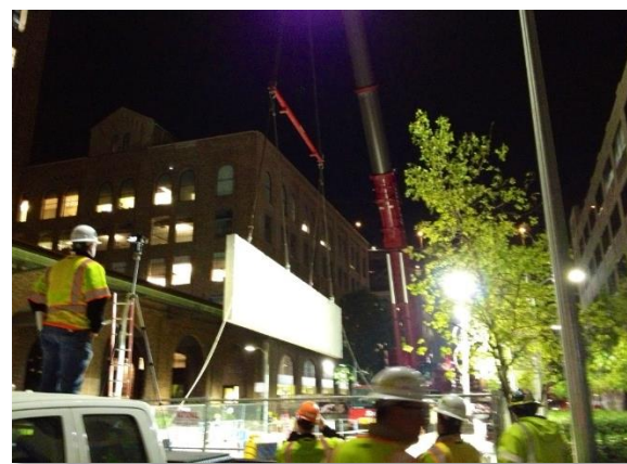
Figure 20. Setting wall in vault with crane, April 1, 2015
