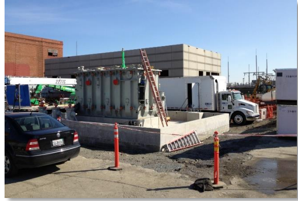
Figure 14. Reactor pad installed, dress and test, February 24, 2016
