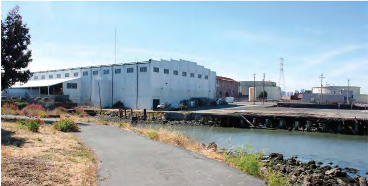
7. Warm Water Cove Park looking northwest
