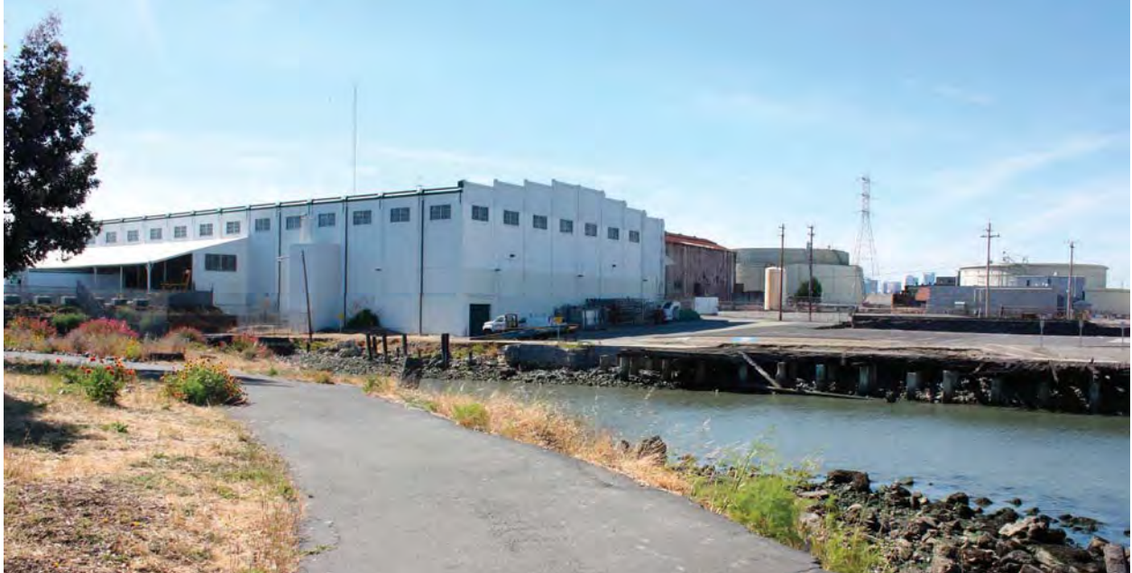
7. Warm Water Cove Park looking northwest
