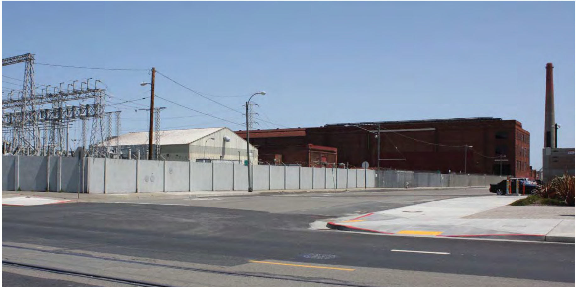
View from 23rd Street at Illinois Street looking northeast (VP 2)
