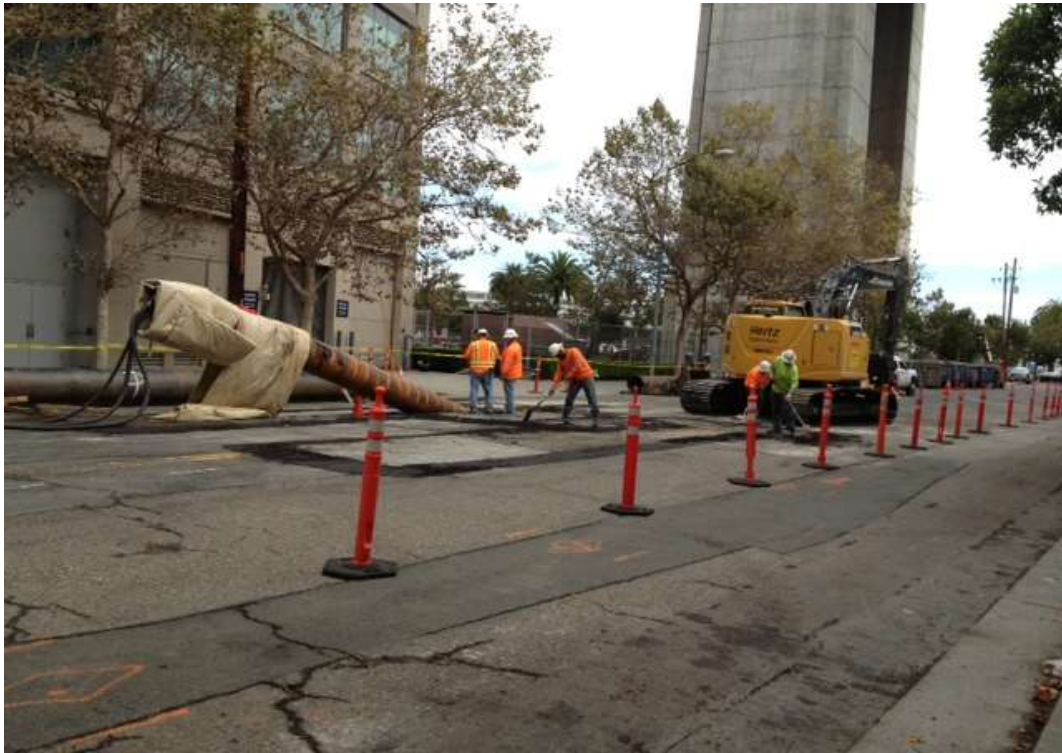
Figure 1 – HDD work activities on Spear Street. View northeast, September 18, 2014.
