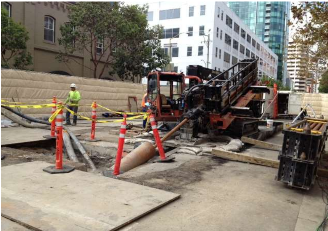
Figure 2 – HDD set-up at Bore #3 on Spear Street. View west, September 29, 2014.
