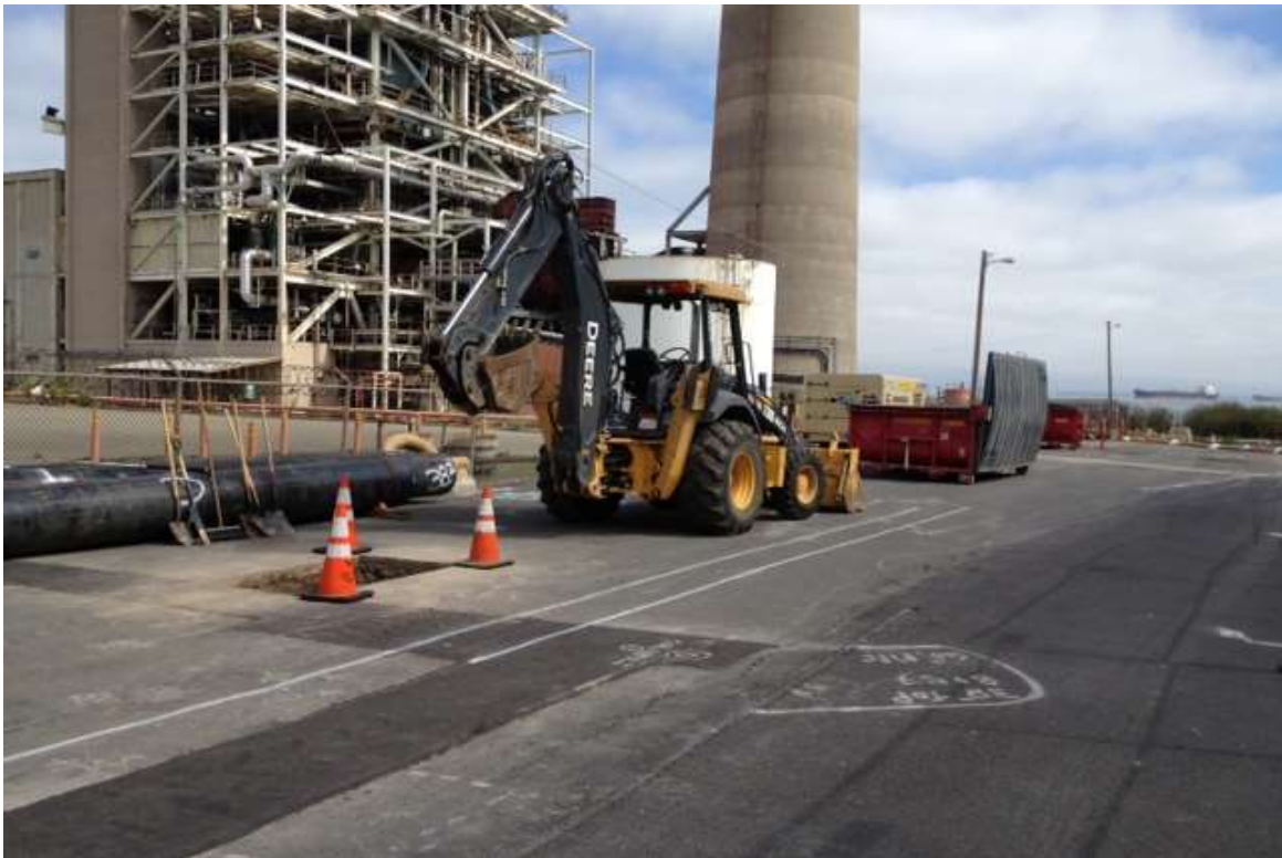
Figure 4 – Water line work on 23 rd Street. View east, September 29, 2014.
