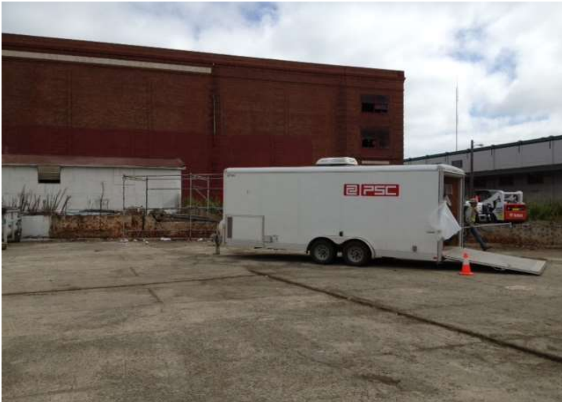
Figure 1 – PSC working on debris clean-up at Potrero Switchyard. View southeast, September 29, 2014.
