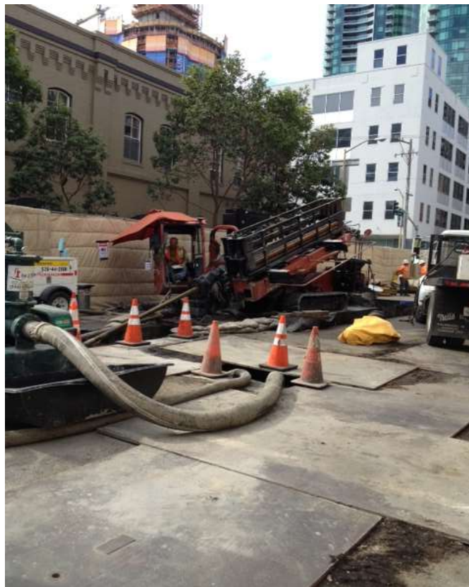
Figure 2 – HDD set-up at Bore #2 on Spear Street. View west, October 16, 2014.
