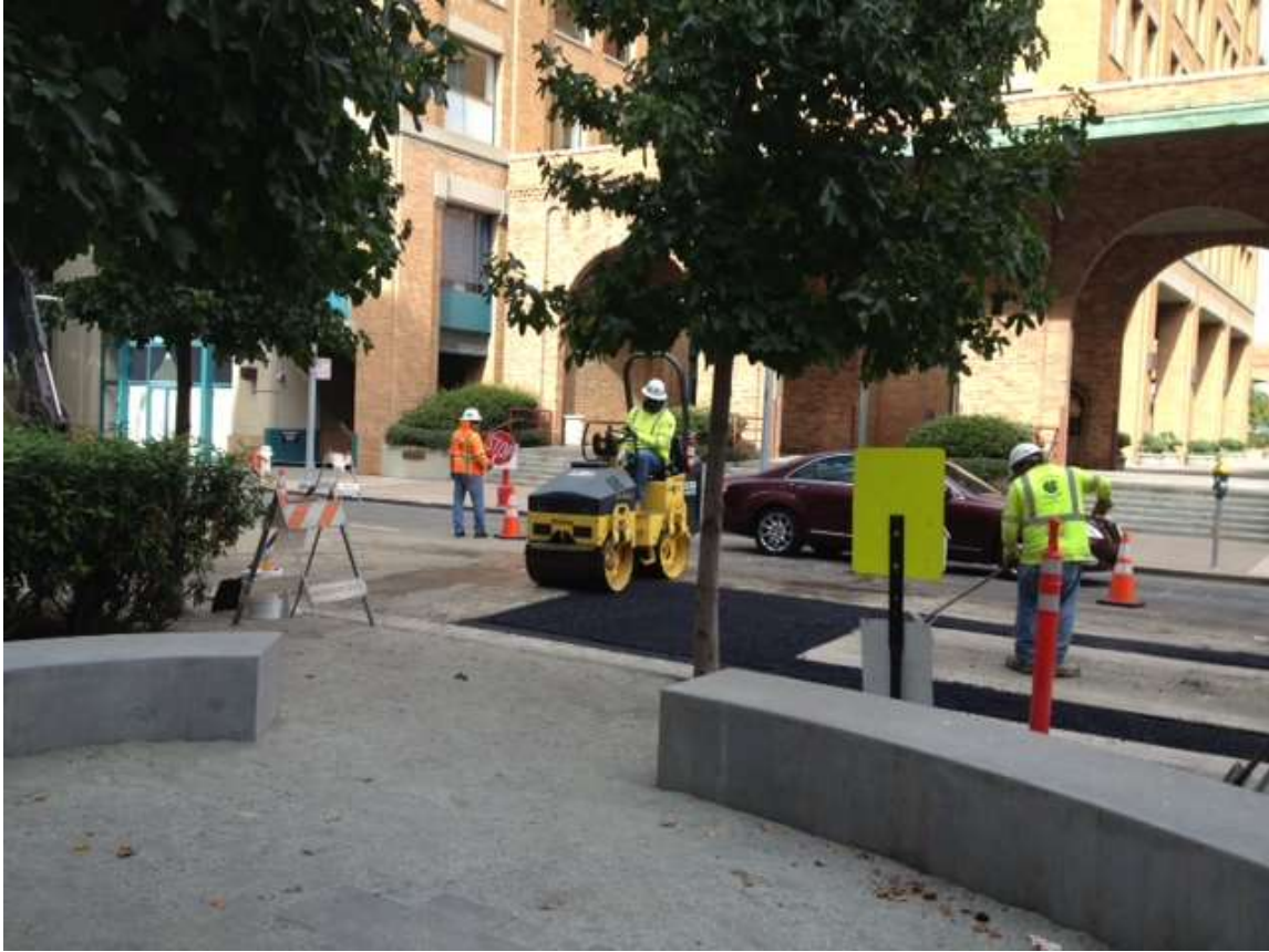
Figure 3 – AT&T fiber optic cable relocation on Spear Street. View north, October 16, 2014.
