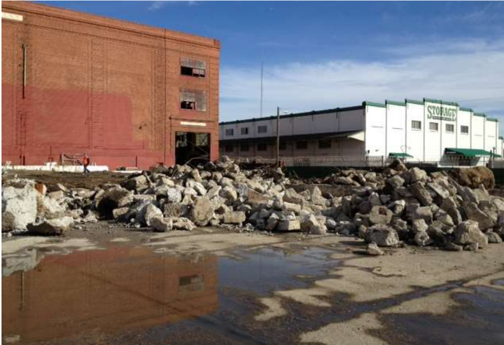
Figure 1 – Demolition of foundations at Potrero Switchyard. View southeast, October 16, 2014.
