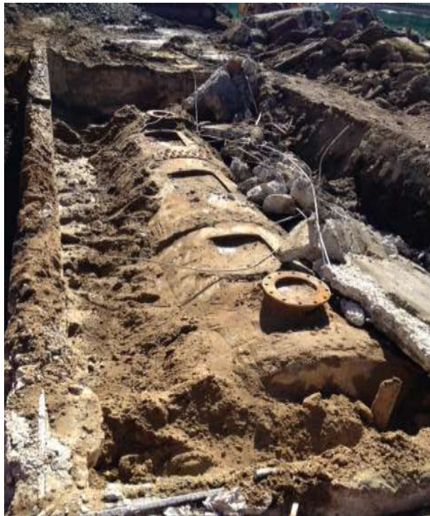
Figure 2 – Underground "condensate" tank uncovered at the Potrero Switchyard. View south, October 21, 2014.
