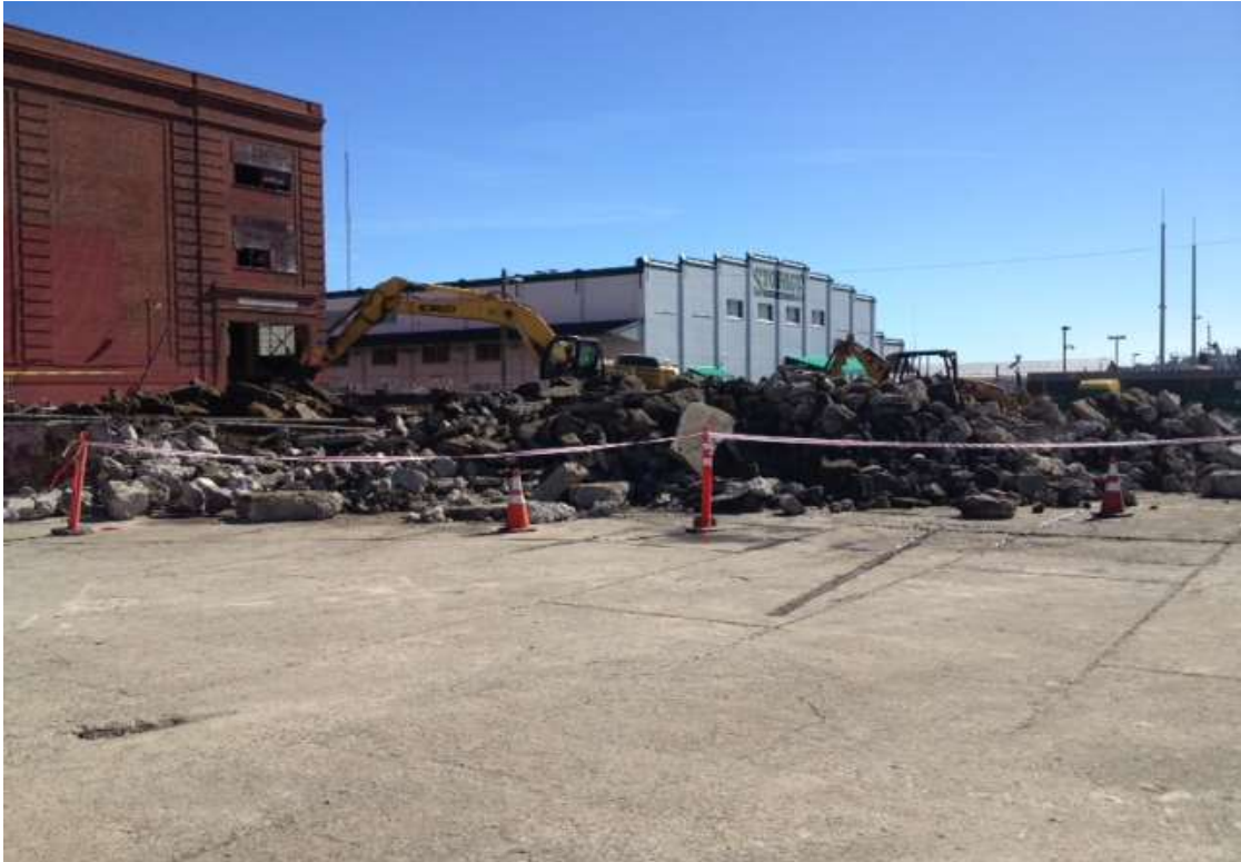
Figure 1 – Demolition of foundations at Potrero Switchyard. View south, October 21, 2014.
