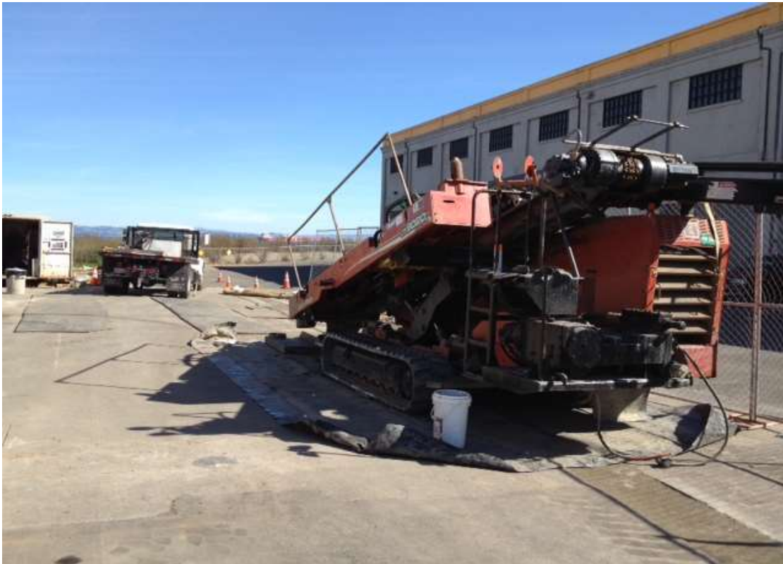
Figure 3 – HDD equipment being staged at 23 rd Street. View east, October 21, 2014.
