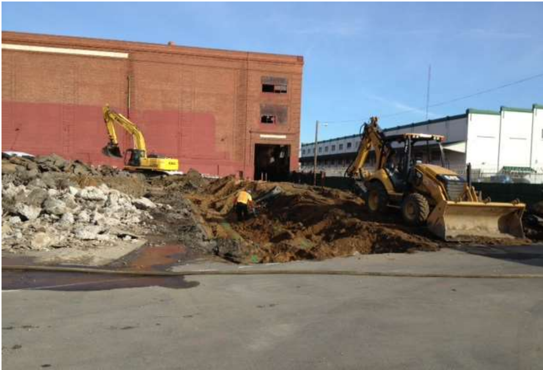
Figure 1 – Demolition of foundations at Potrero Switchyard. View east, November 3, 2014.
