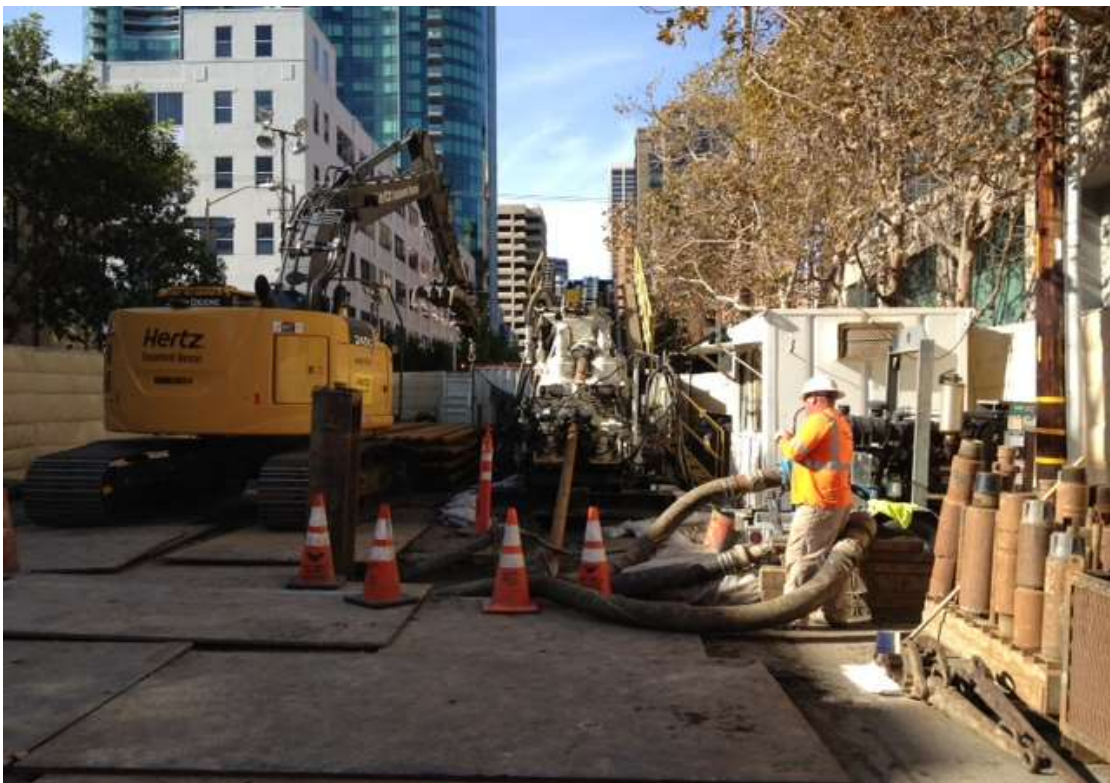
Figure 2 – HDD set up on Spear Street. View west, November 3, 2014.
