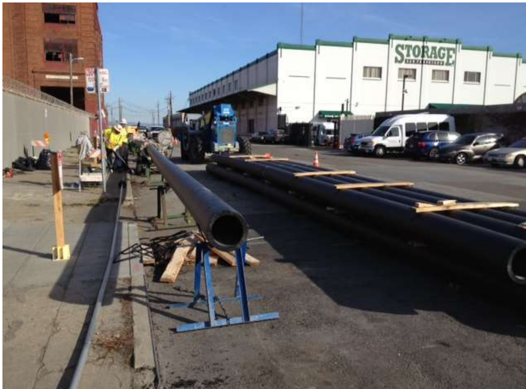
Figure 4 –Fusing HDPE 12-inch pipe on 23 rd Street. View east, November 3, 2014.
