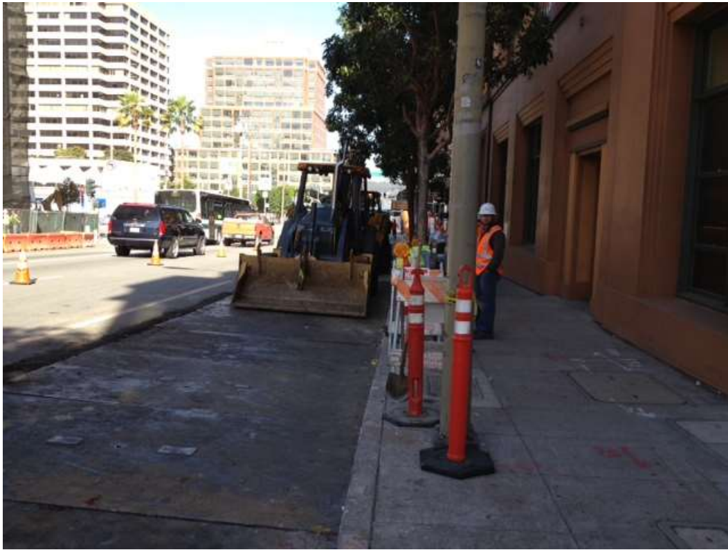
Figure 5 – Trenching activities on Folsom Street. View north, November 3, 2014.
