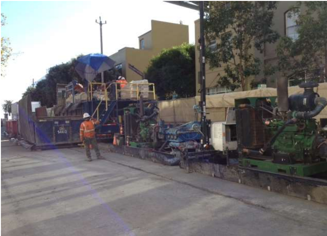
Figure 3 – Additional HDD equipment set-up on Spear Street. View southeast, November 3, 2014.
