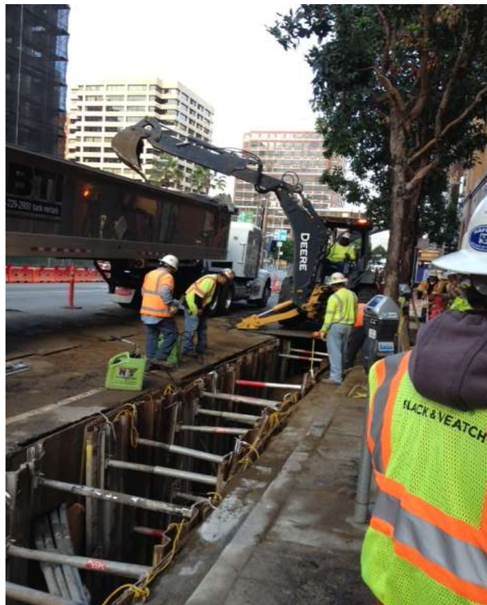
Figure 4 –Excavation work on Folsom Street. View north, November 13, 2014.
