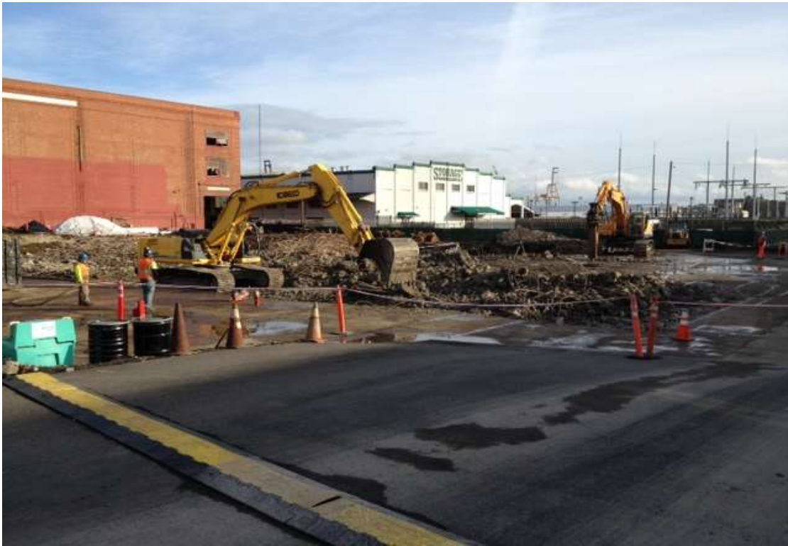
Figure 1 – Demolition of foundations at Potrero Switchyard. View southeast, November 13, 2014.
