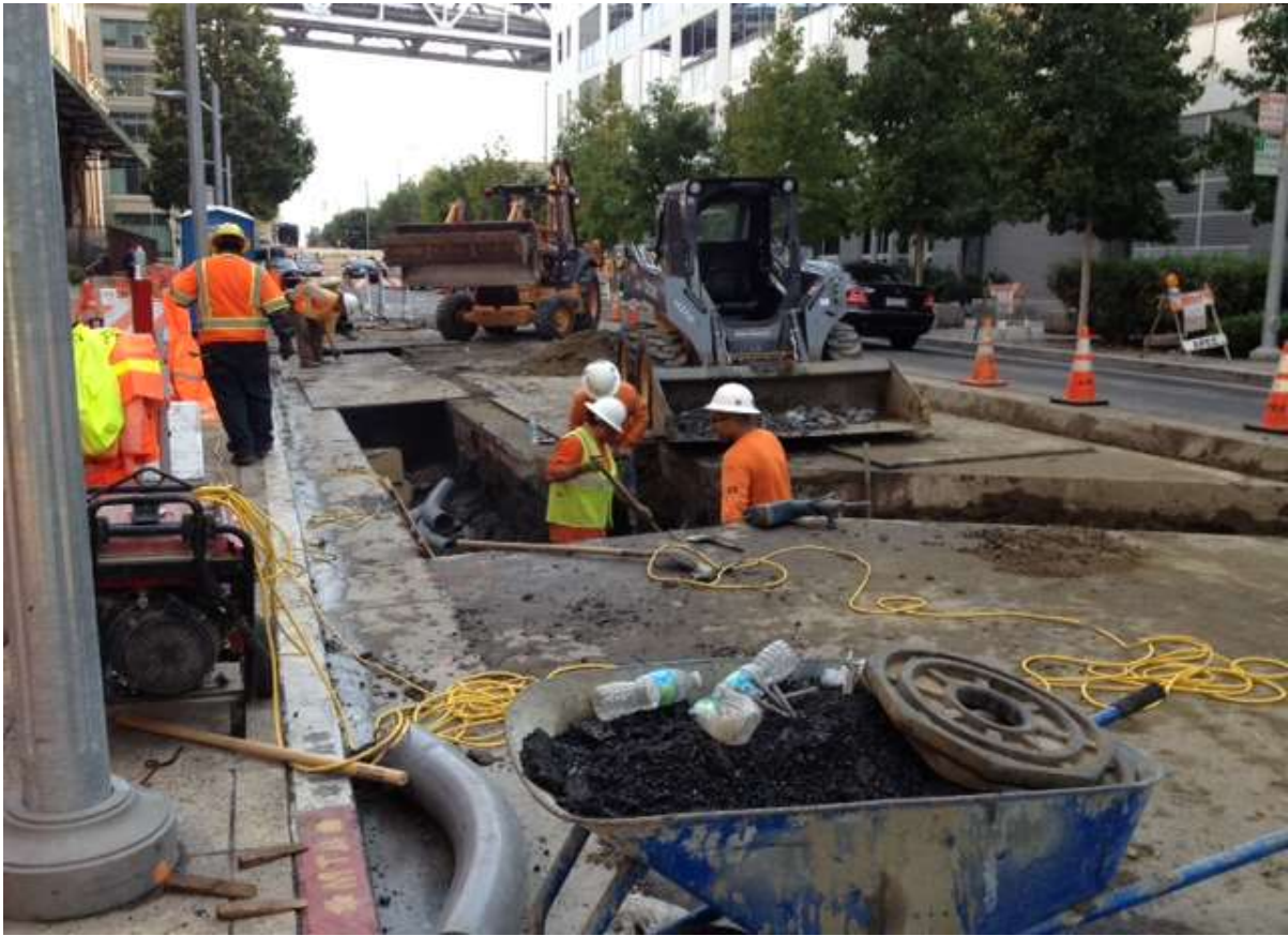
Figure 5 – 12 kV relocation activities on Spear Street. View east, November 13, 2014.
