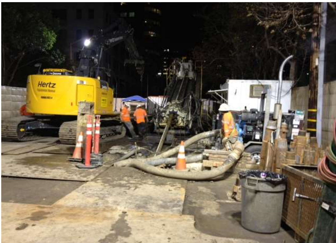
Figure 2 – HDD night work on Spear Street. View west, November 13, 2014.
