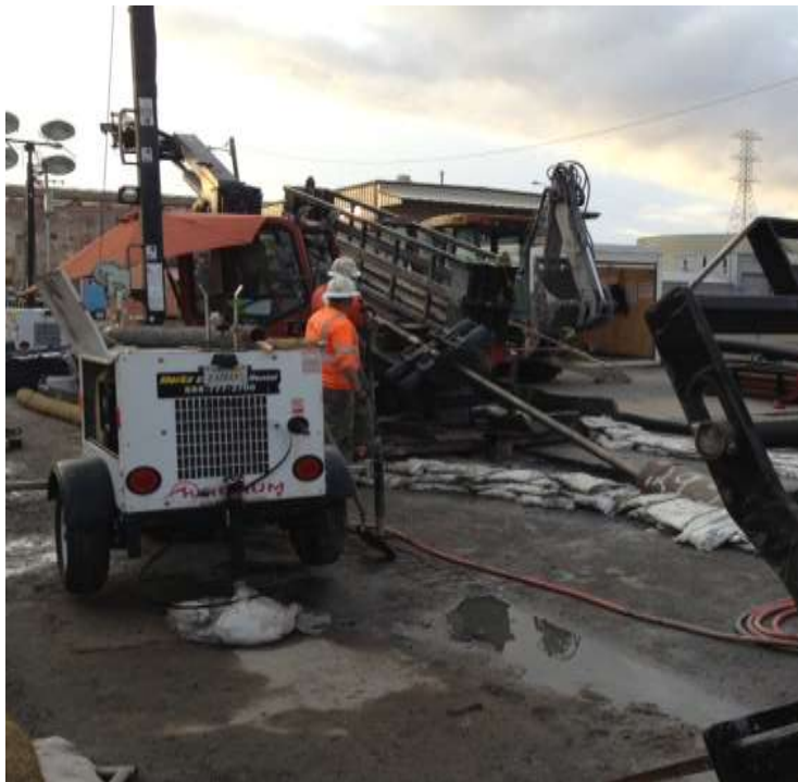
Figure 3 – HDD South on 23 rd Street. View west, November 13, 2014.
