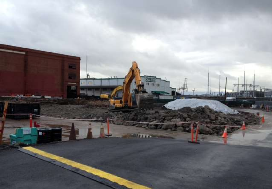
Figure 1 – Demolition of foundations at Potrero Switchyard. View southeast, November 20, 2014.
