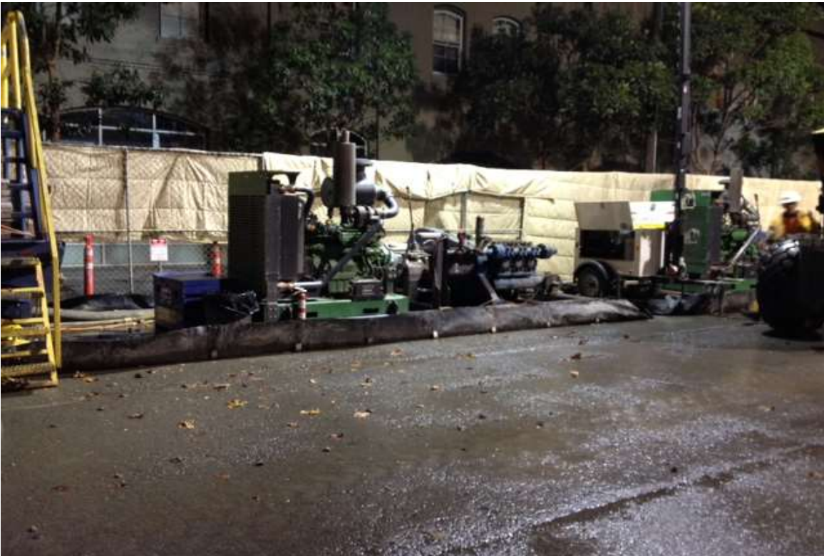
Figure 2 – HDD night work on Spear Street. View south, November 20, 2014.
