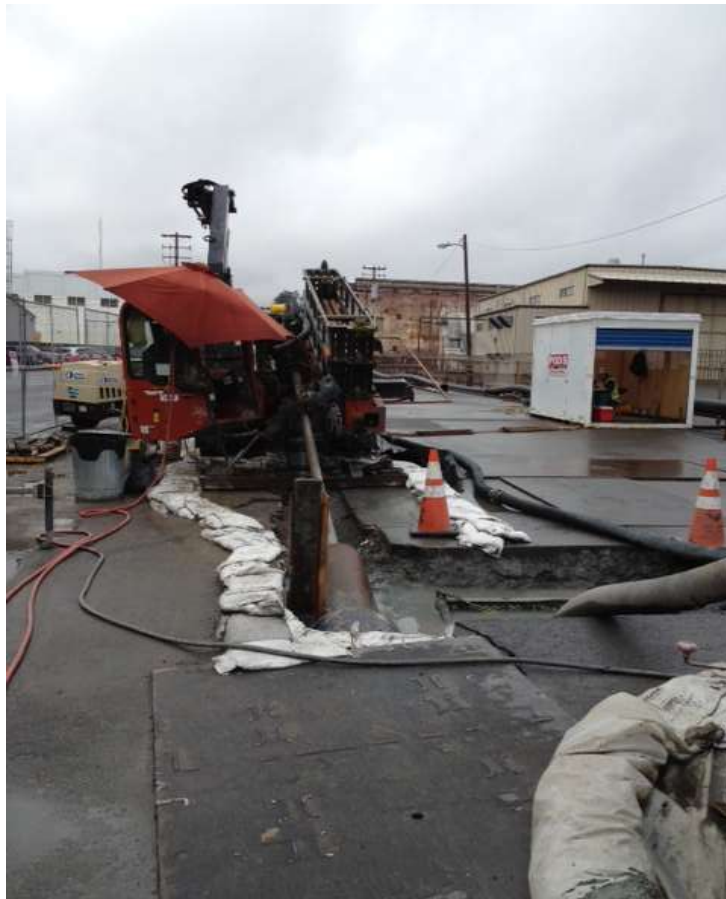
Figure 3 – HDD South on 23 rd Street. View west, November 20, 2014.
