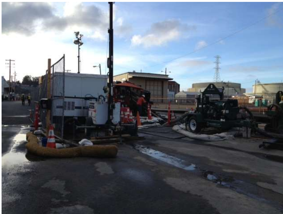
Figure 4 – HDD South operations. View west, December 4, 2014.
