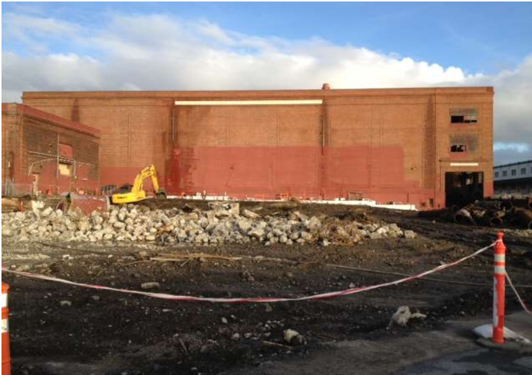
Figure 1 – Demolition and excavation at Potrero Switchyard, View east, December 4, 2014.
