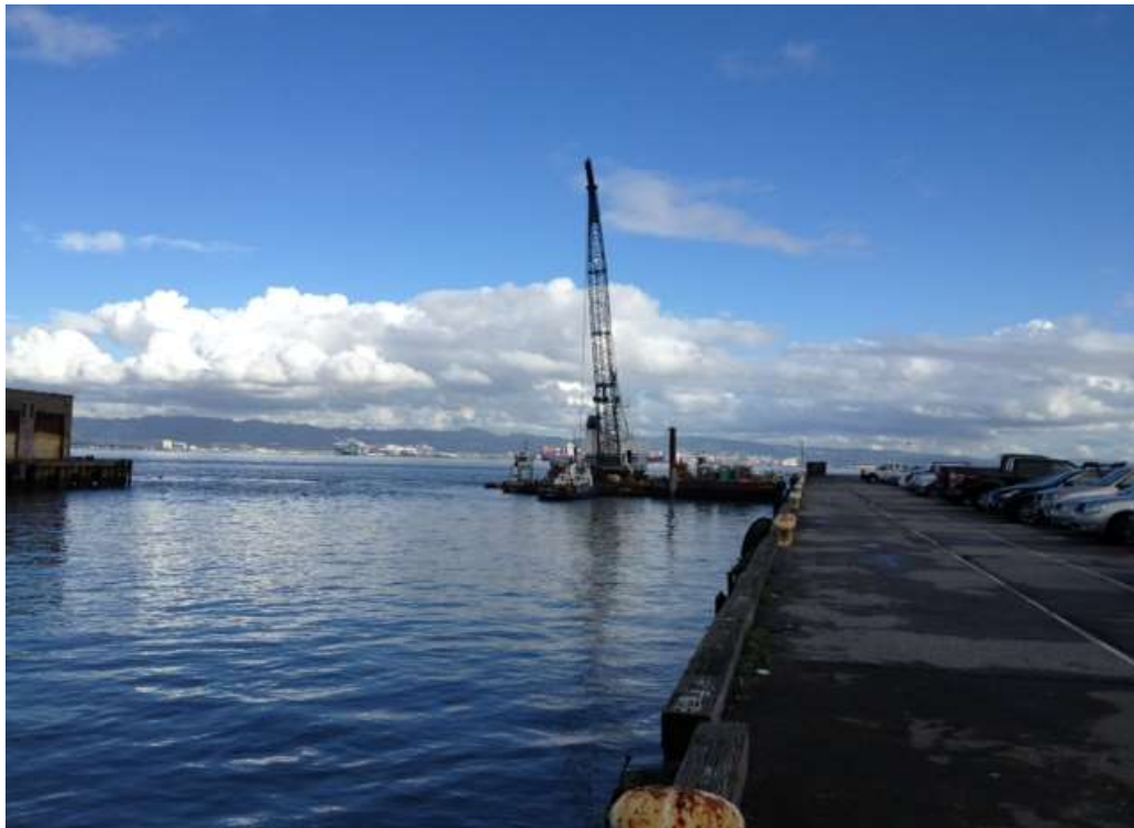
Figure 2 – Vortex set-up at HDD North receiving pit. View east, December 4, 2014.
