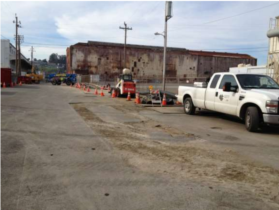
Figure 5 – Underground duct bank trench area on 23 rd Street. View west, January 5, 2015.
