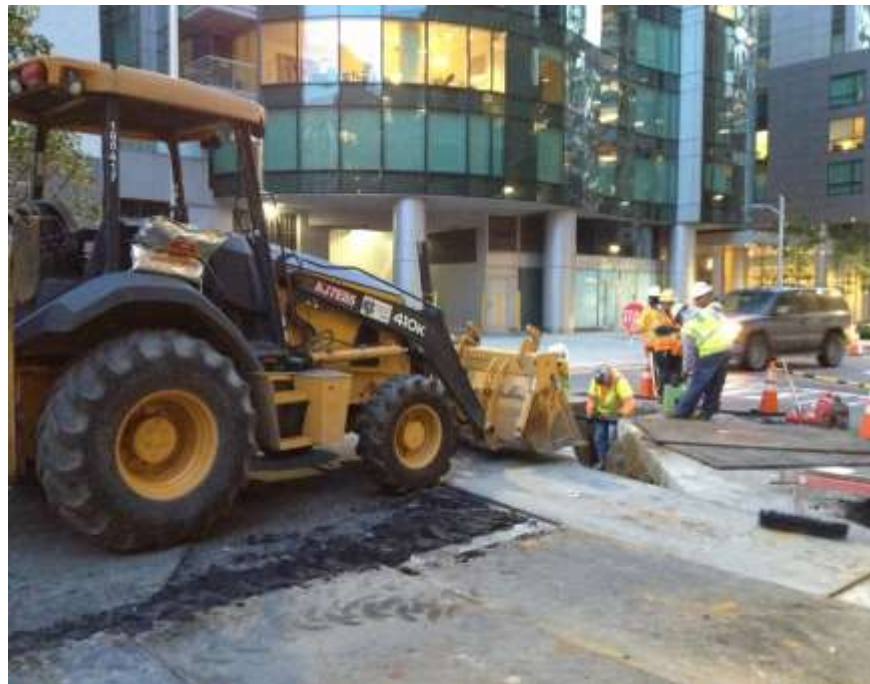
Figure 4 – Shoring trench excavation on Spear Street. View west, January 5, 2015.
