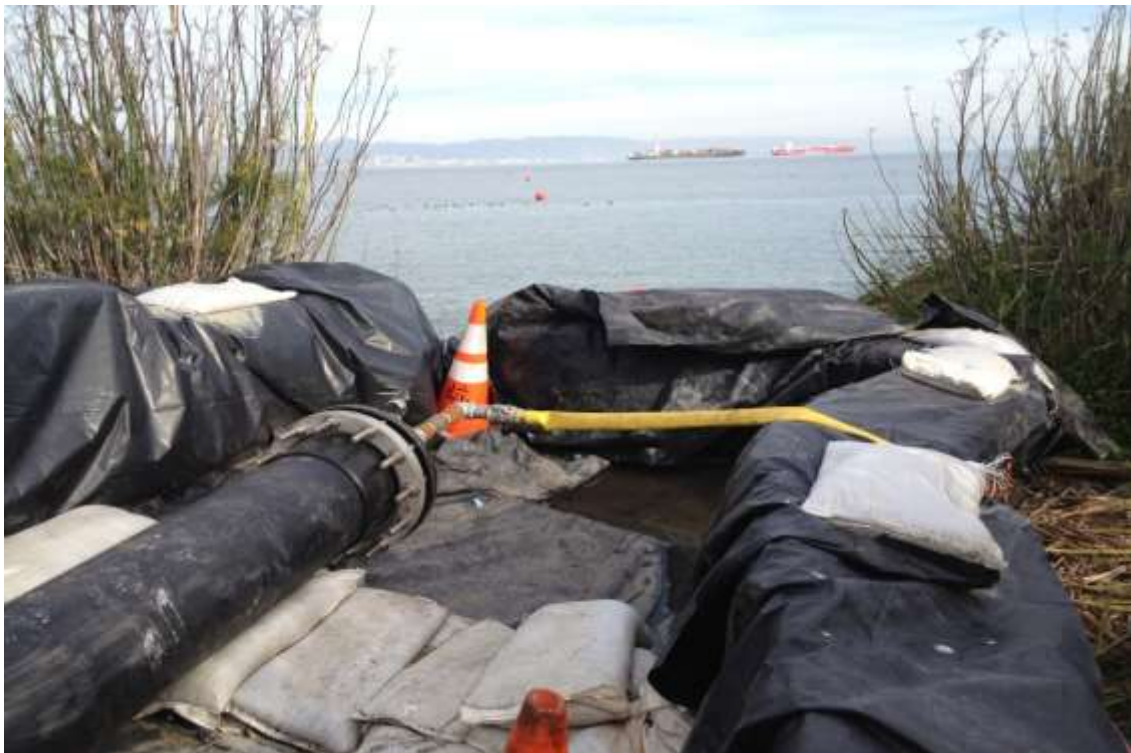
Figure 2 – Hydrotest of HDPE pipe at HDD South. View east, January 5, 2015.
