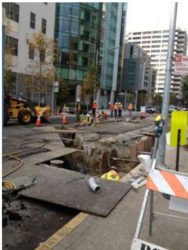
Figure 4 – Utility relocation work on Spear Street. View west-southwest, January 15, 2015.
