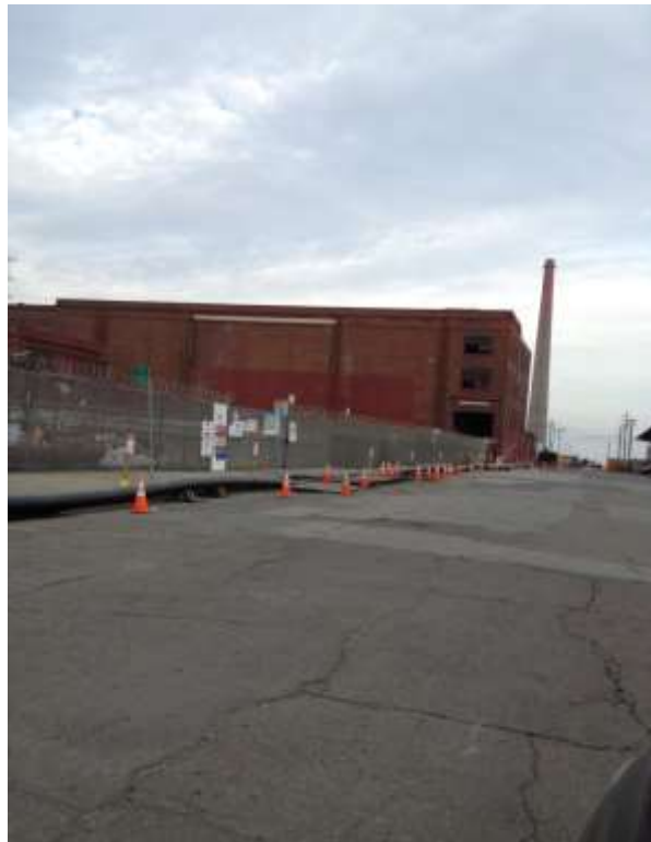
Figure 2 – HDPE pipe staged along 23 rd Street for hydrotesting. View east, January 15, 2015.
