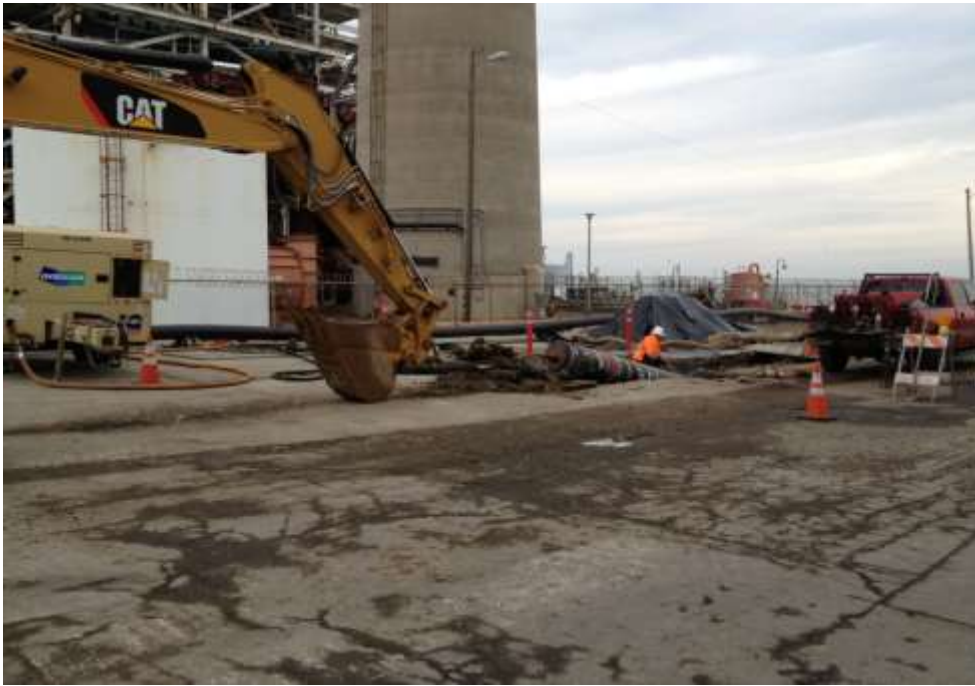
Figure 1 – Crews removing drill casing at HDD South. View east-northeast, January 15, 2015.
