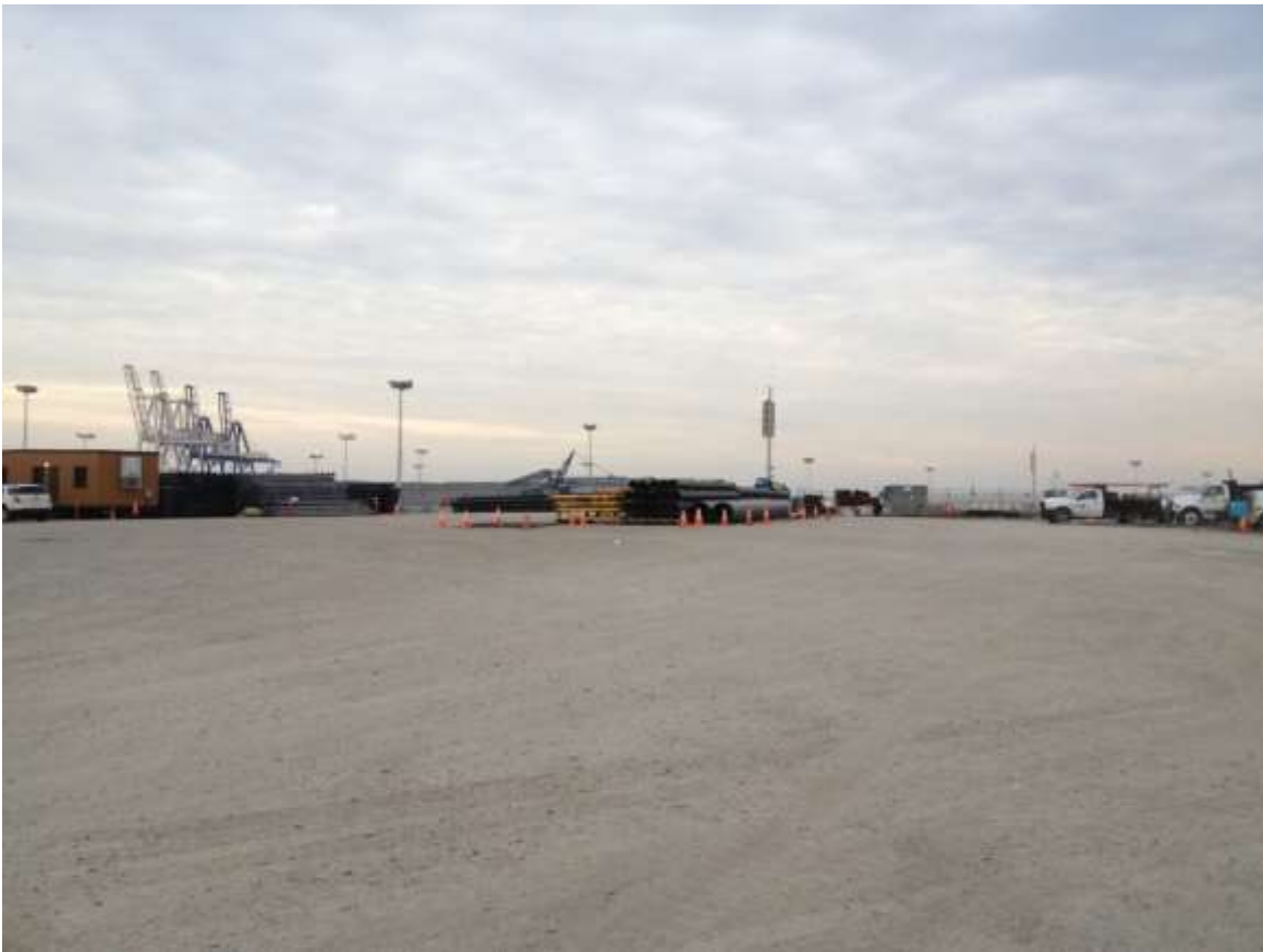
Figure 5 – Staging equipment and materials at Amador Yard. View south, January 15, 2015.
